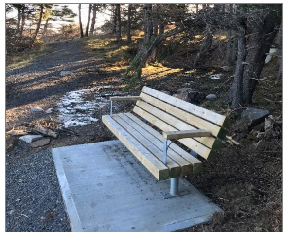
Bench repairs at Breaker’s Park
