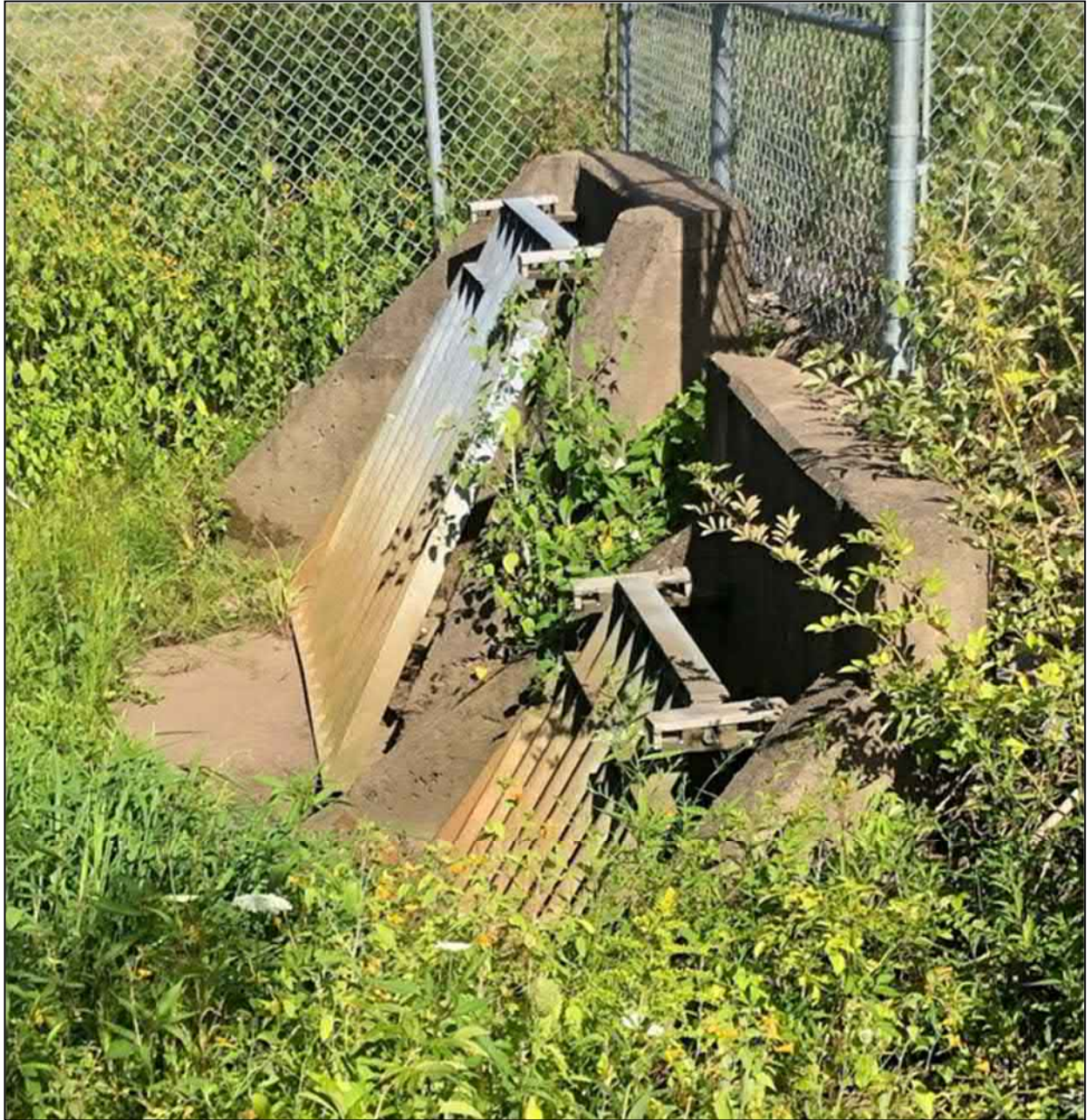
Figure 4-4: Culvert Inlets to Cole Harbour Road
