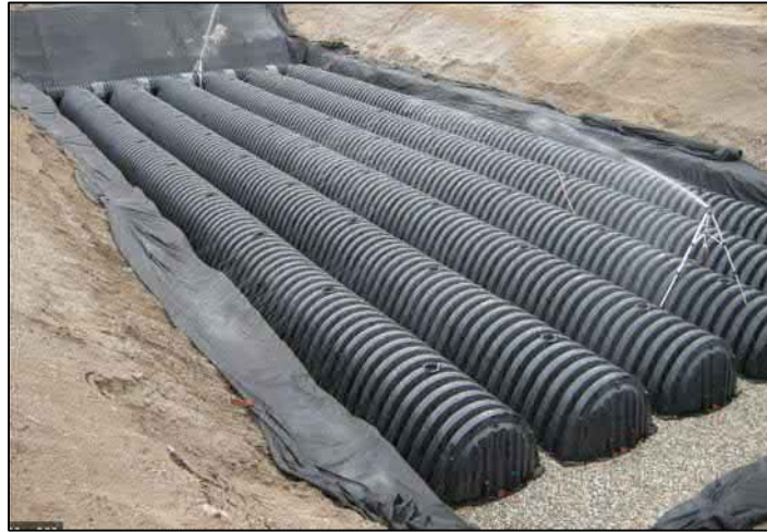
Figure 4-6: Example of HDPE Detention Chambers ( https://www.conteches.com )
