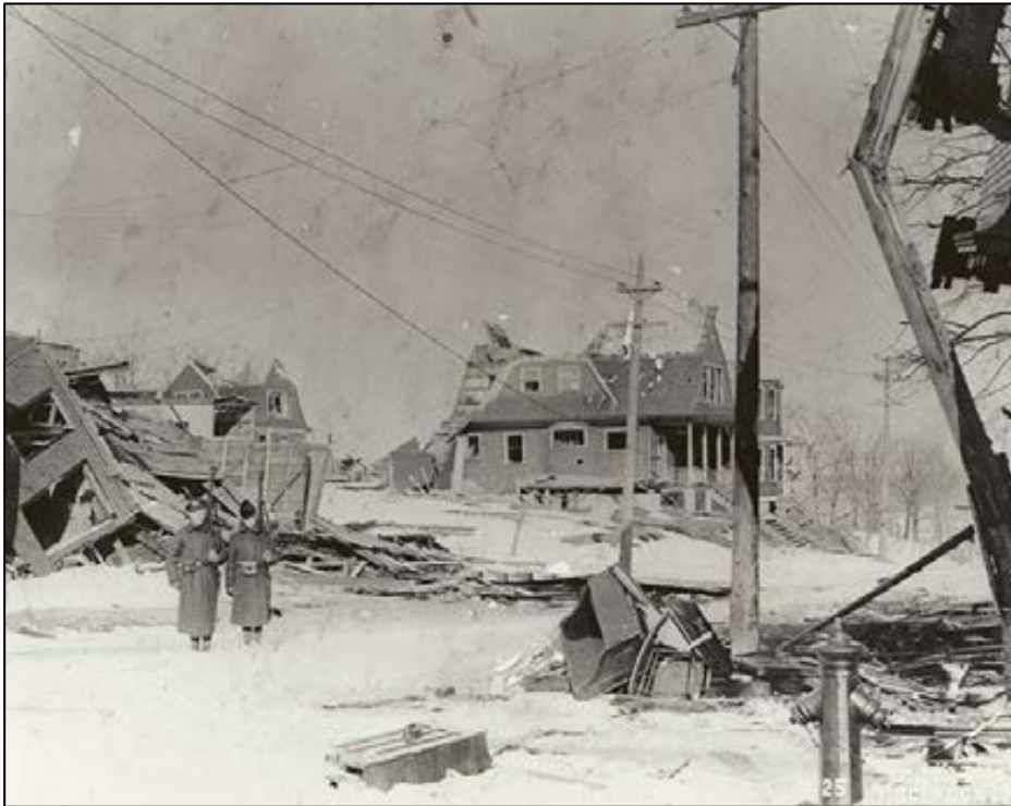
Kaye Street after the Halifax Explosion
