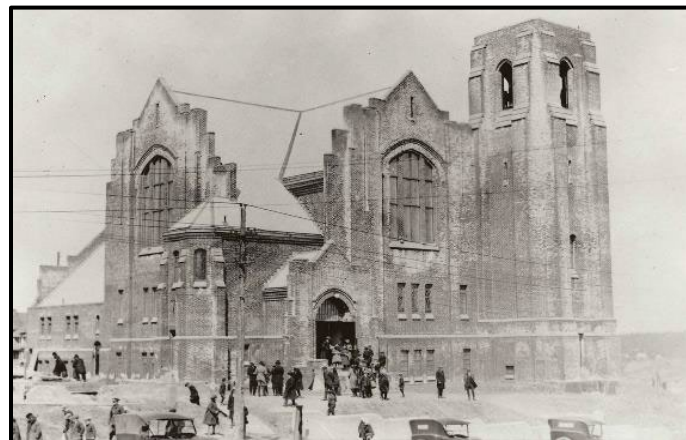
United Memorial Church shortly after completion, 1921
