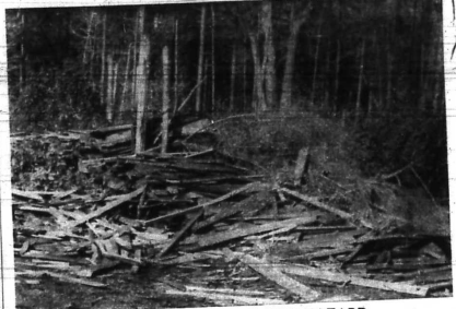
DEBRIS MARS SCENE, IS FIRE HAZARD
