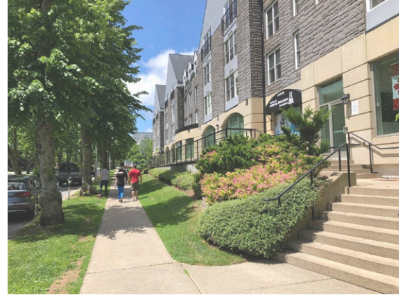
Figure 4.3.2: Appropriate Institutional Setback. Approximately 4.0 m from the streetline and comprised of vegetation and entrances.
