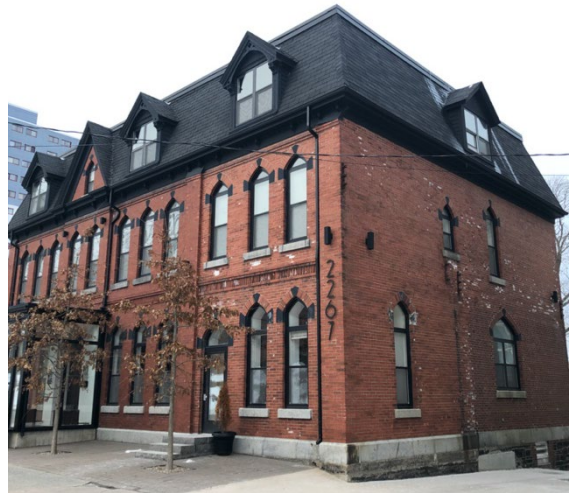
Façade and south wall of St. Patrick's rectory in February 2020 (Swaffer, 2020)
