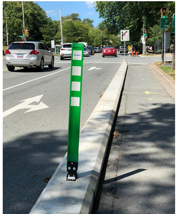
Figure A-2: Pre-Cast Concrete Curb and Flexible Bollard, South Park Street, Halifax,
