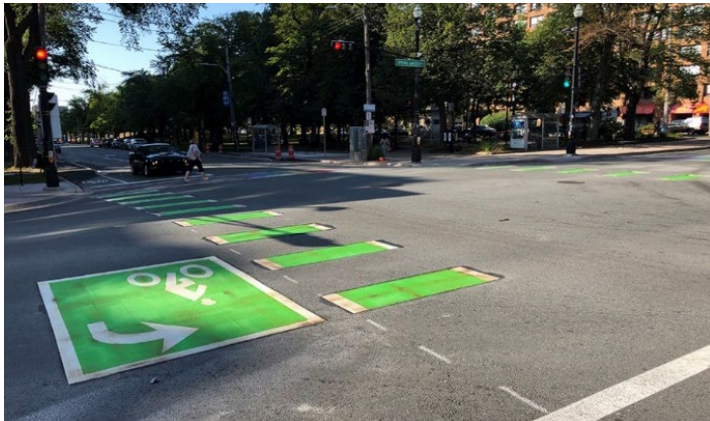
Figure A-4: Example of Bikeway Intersection Markings, South Park Street, Halifax, NS
