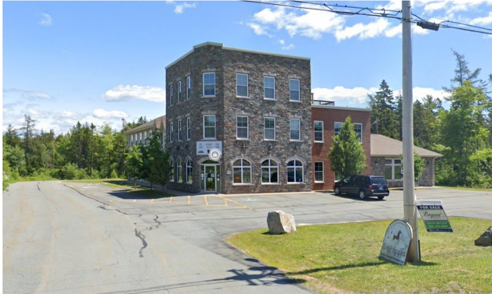
Street view of existing building
