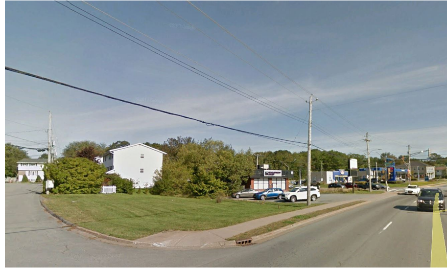
Looking north towards subject site from Malik Court and Cobequid Road intersection
