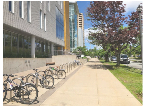
Figure 4.3.4: Appropriate Institutional Setback. Approximately 4.0 m from the streetline and comprised of vegetation, an extended sidewalk, bicycle racks, and entrances.
