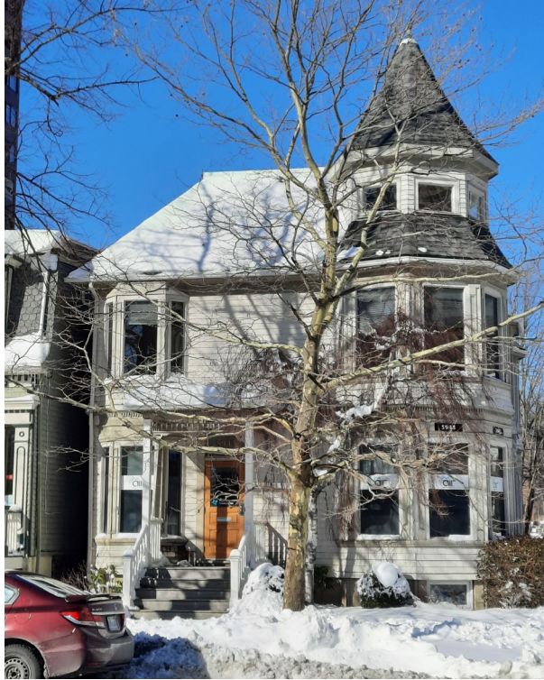
Figure 8: South façade of 5943 Spring Garden Road (09 February 2021)
