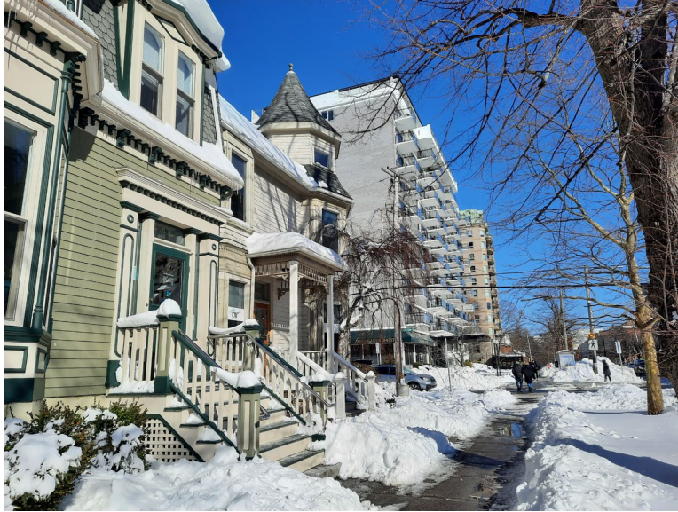
Figure 19: 5945 and 5943 Spring Garden Road, with Spring Garden Terrace visible to the right (09 February 2021)
