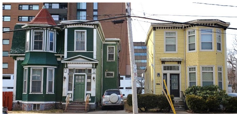
Figure 2: 1538 and 1540 Carlton Street in early spring 2020
