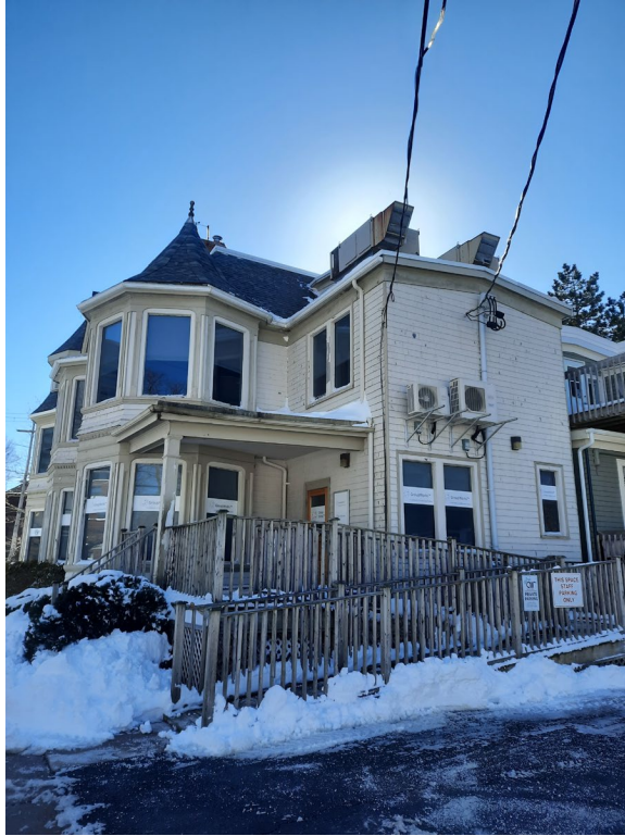
Figure 10: North and east façades of 5943 Spring Garden Road (09 February 2021)
