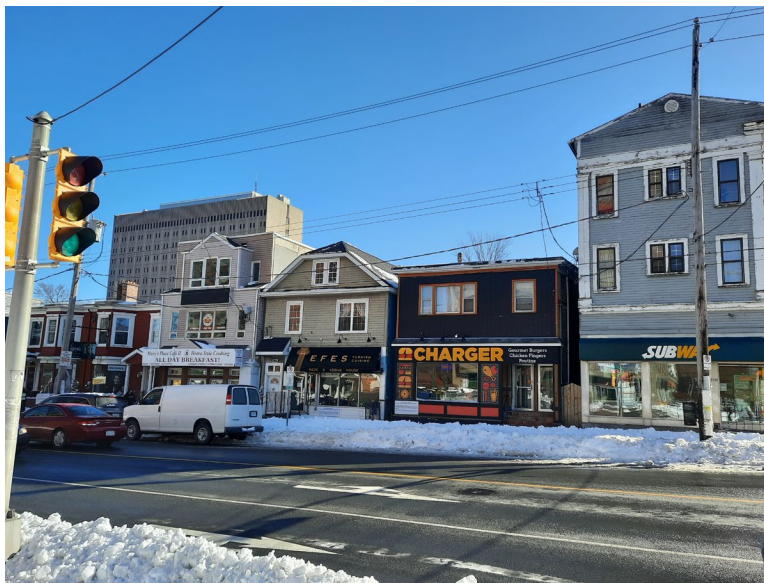
Figure 20: West portion of buildings to be demolished as part of Case 20218 (09 February 2021)
