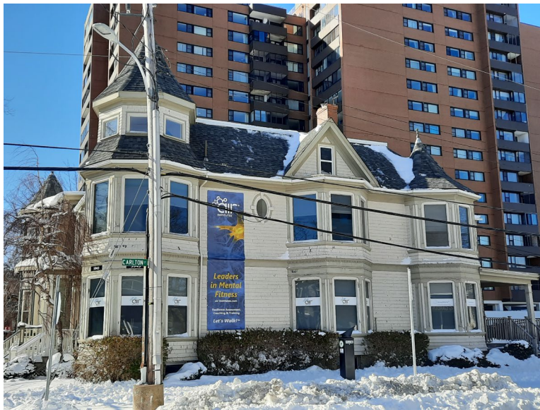
Figure 9: East façade of 5943 Spring Garden Road (09 February 2021)
