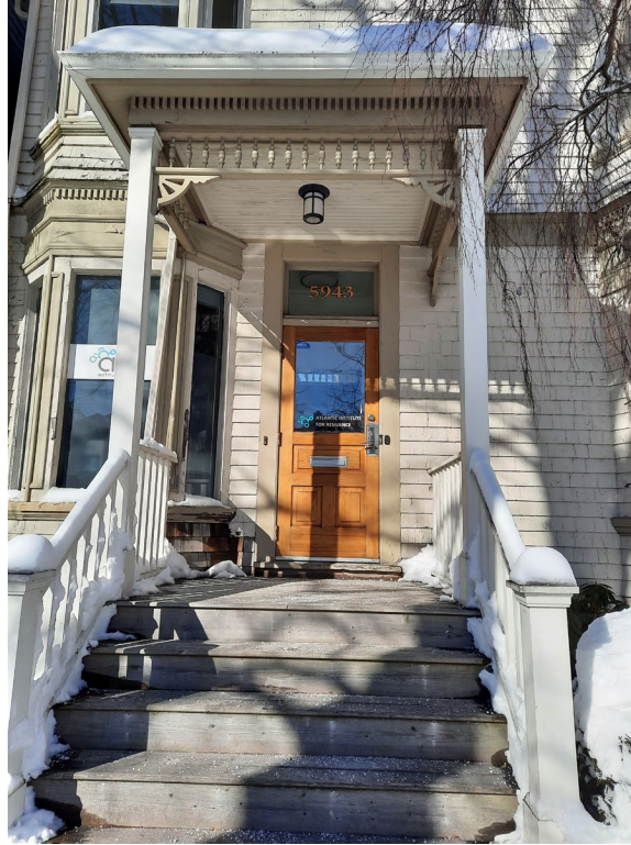
Figure 12: Main entrance to 5943 Spring Garden Road (09 February 2021)
