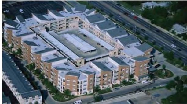
Preferred: parking integrated internal to block development, hidden behind ‘sleeves’ of active uses
