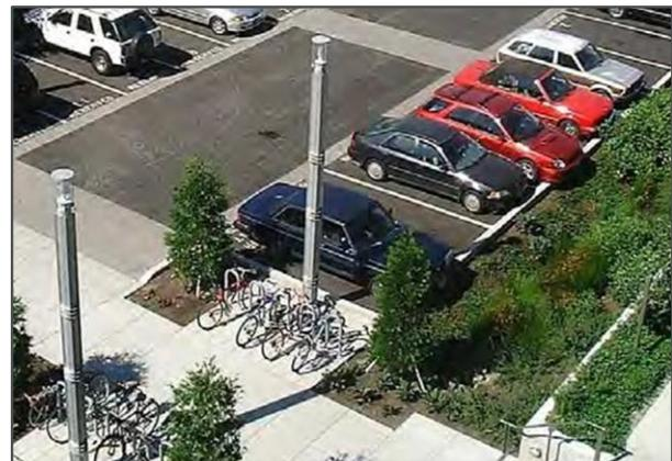
Surface runoff from parking is treated by vegetated system
