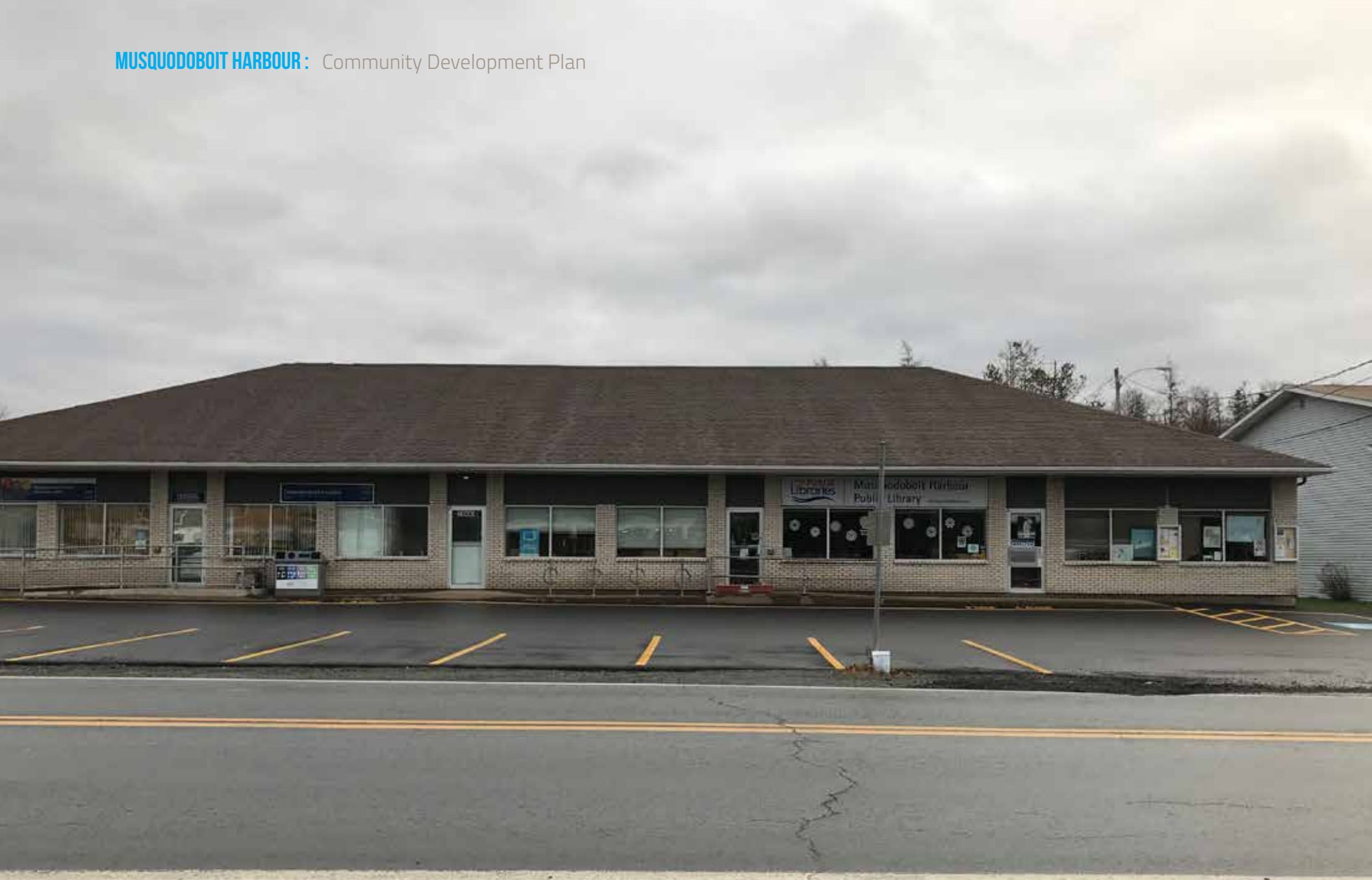
FIGURE 49. Typical Marine Drive today
