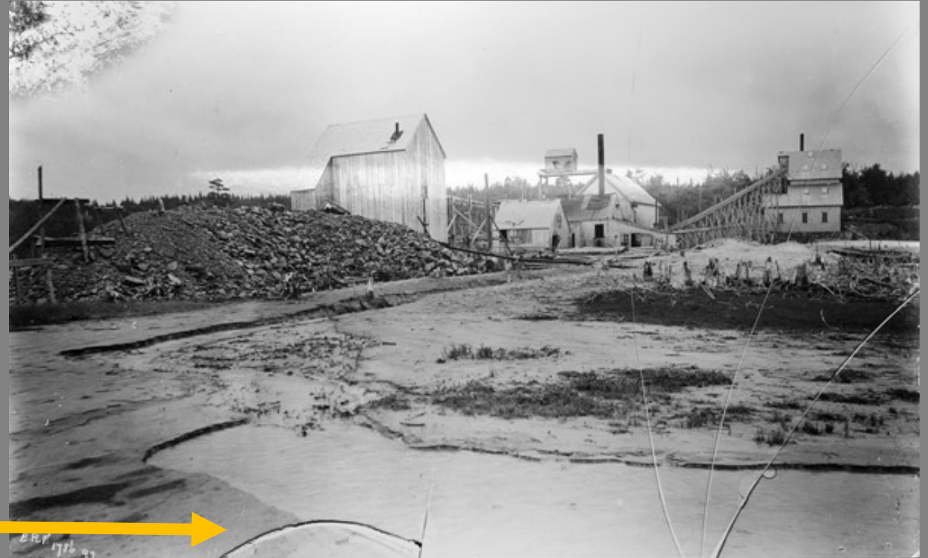
Stamp mill engine house and shaft house, Mooseland Gold Mining Co., 1897. Historical Photograph by E. R. Faribault. Geological Survey of Canada Photo #5297.
