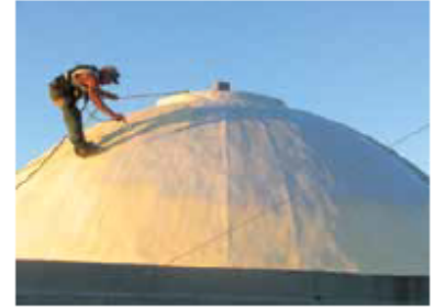
The dome of Melville City Hall was originally an uninsulated, painted-metal covering that caused persistent condensation problems. Applying insulating polyurethane foam with aluminized coating was a cost-effective solution that was compatible with the historic metallic look of the dome. If a more elaborate solution is contemplated in the future, the polyurethane could be removed.
