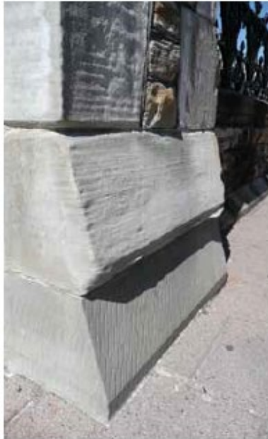
The new pieces of stone on the Wellington Wall at the Parliament Grounds in Ottawa are clearly visible on close inspection due to a different tooling technique.
