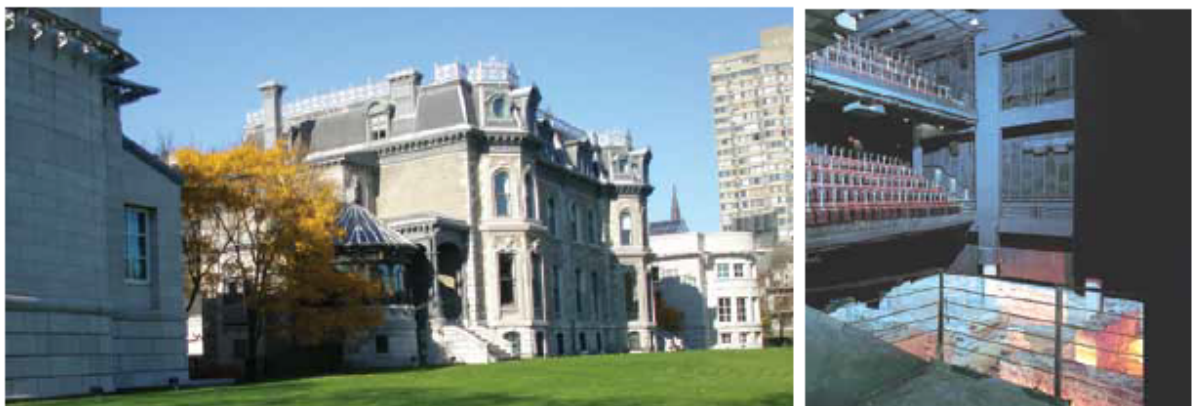
These two additions in Montreal show the range of possibilities for successful additions to historic places. Although the addition to Shaughnessy House by the Canadian Centre for Architecture has a larger footprint than the original building, it demonstrates a subtle approach, using compatible scale, proportions of openings, materials and details, which acknowledges the original building. Pointe-à-Callière Museum of Archaeology and History illustrates a contrasting contemporary approach where an archaeological site has been successfully integrated into a new design in ways that communicate the site's heritage value.
