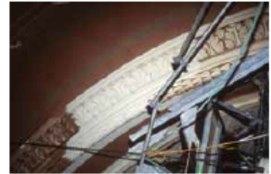
When restoring decorative plaster in the Walker Theatre in Winnipeg, moulds were made of existing plaster elements. The deteriorated plaster was then patched and repaired using the moulds to match the original.
