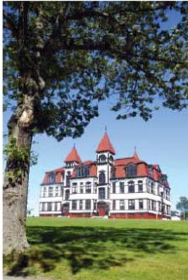
Despite changing requirements in education, the Lunenburg Academy in Nova Scotia remains in its original building and setting. The Academy was designed using green space, natural lighting and ventilation in a way that is still valid for school use today.
