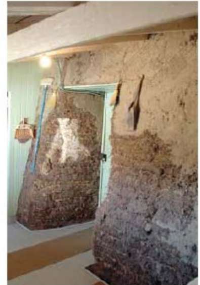
The lean-to is a character-defining element that shows the evolution of the Addison Sod House in Saskatchewan from a rustic sod dwelling to a comfortable home. Removing the later changes to restore the house to an earlier period would not be appropriate because it would remove elements that have heritage value.
