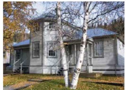
This Dawson City building, originally built to be the temporary location for the government telegraph office, was rehabilitated into housing units.
