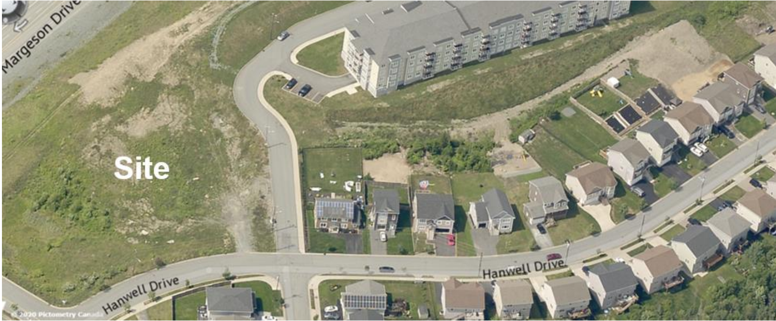
Existing apartment building and houses along Hanwell Dr.
