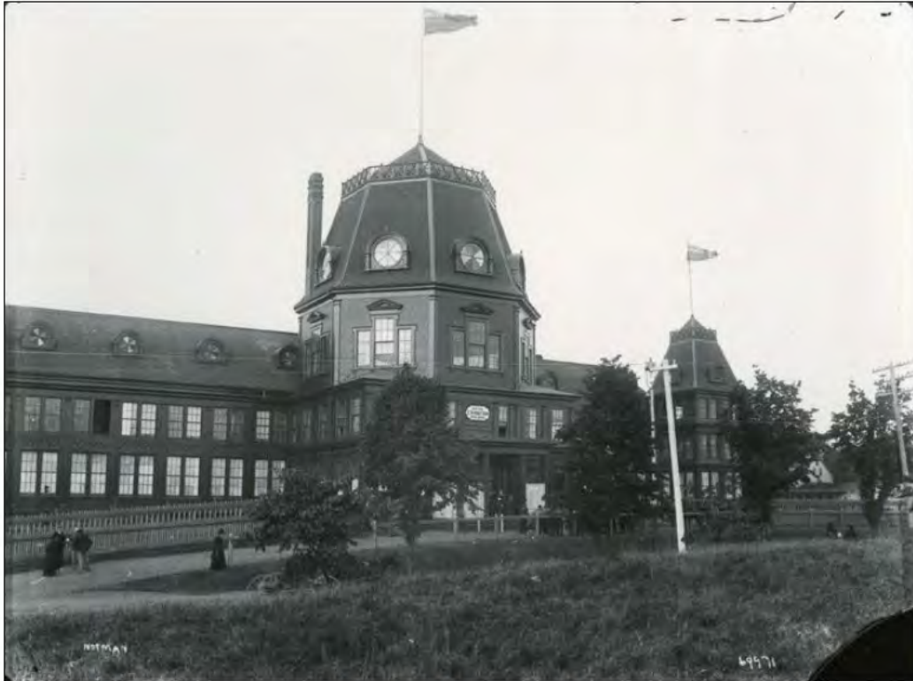
Figure 3.2-50: The exterior of the Exhibition Building on Tower Road. 301
