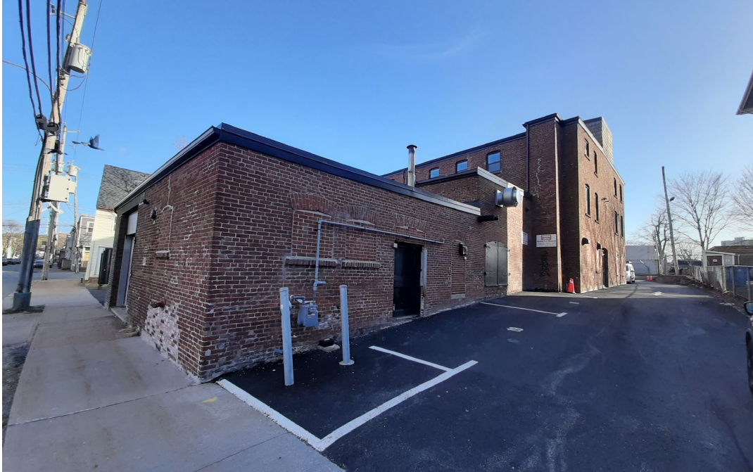
Figure 11: East and north elevations, with the east wing to the left (April 14, 2021)
