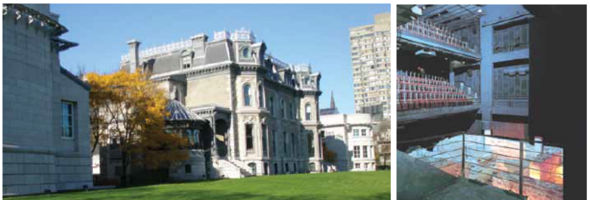
These two additions in Montreal show the range of possibilities for successful additions to historic places. Although the addition to Shaughnessy House by the Canadian Centre for Architecture has a larger footprint than the original building, it demonstrates a subtle approach, using compatible scale, proportions of openings, materials and details, which acknowledges the original building. Pointe-à-Callière Museum of Archaeology and History illustrates a contrasting contemporary approach where an archaeological site has been successfully integrated into a new design in ways that communicate the site's heritage value.
