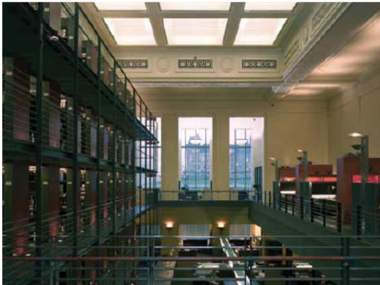
Space to temporarily house the Library of Parliament in the former Bank of Nova Scotia Building on Sparks Street in Ottawa. The entire intervention was designed to be reversible.
