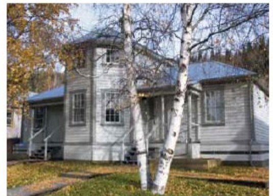
This Dawson City building, originally built to be the temporary location for the government telegraph office, was rehabilitated into housing units.
