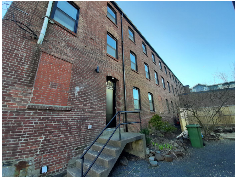
Figure 10: East and south elevations with east wing to the right (April 14, 2021)
