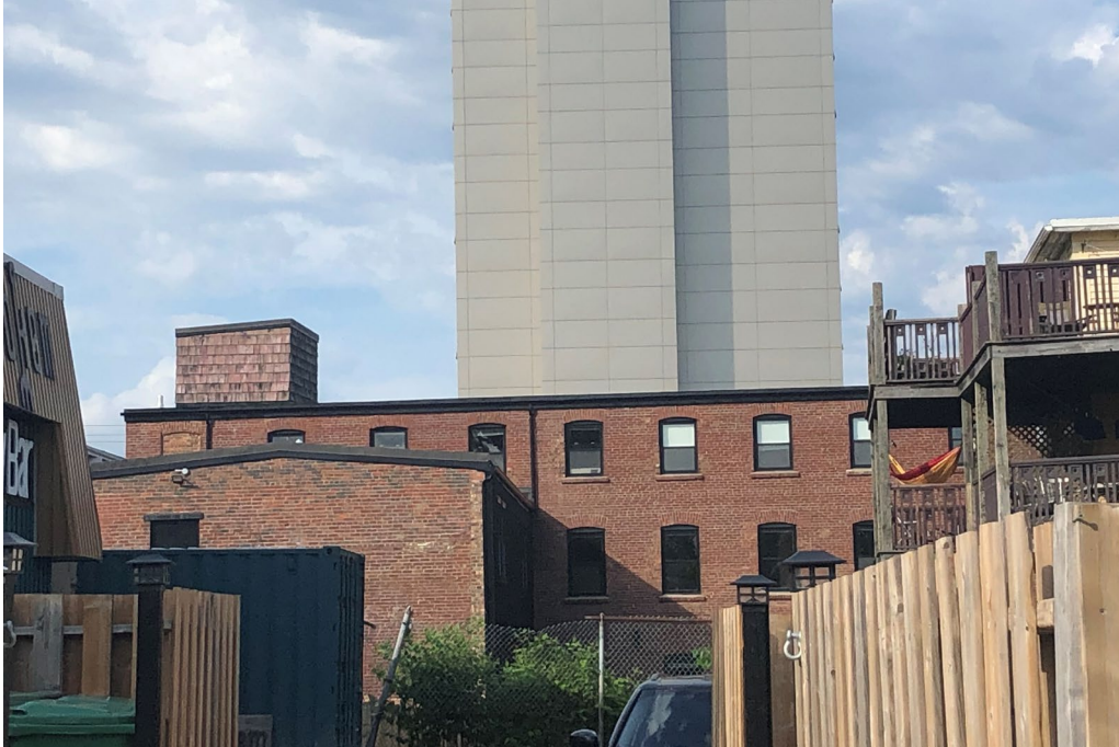
Figure 13: West elevation with the west wing to the left (June 9, 2021)
