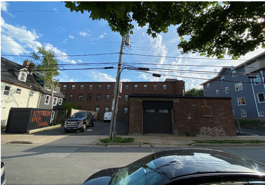
Figure 12: East elevation of the building with east wing to the right (June 9, 2021)
