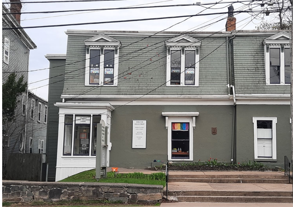
Figure 11: East addition (May 4, 2021)
