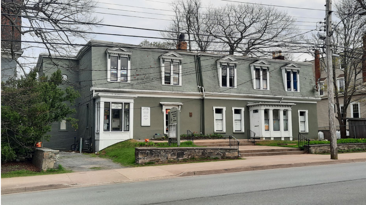
Figure 6: North and east façades of 5500 Inglis Street (May 4, 2021)
