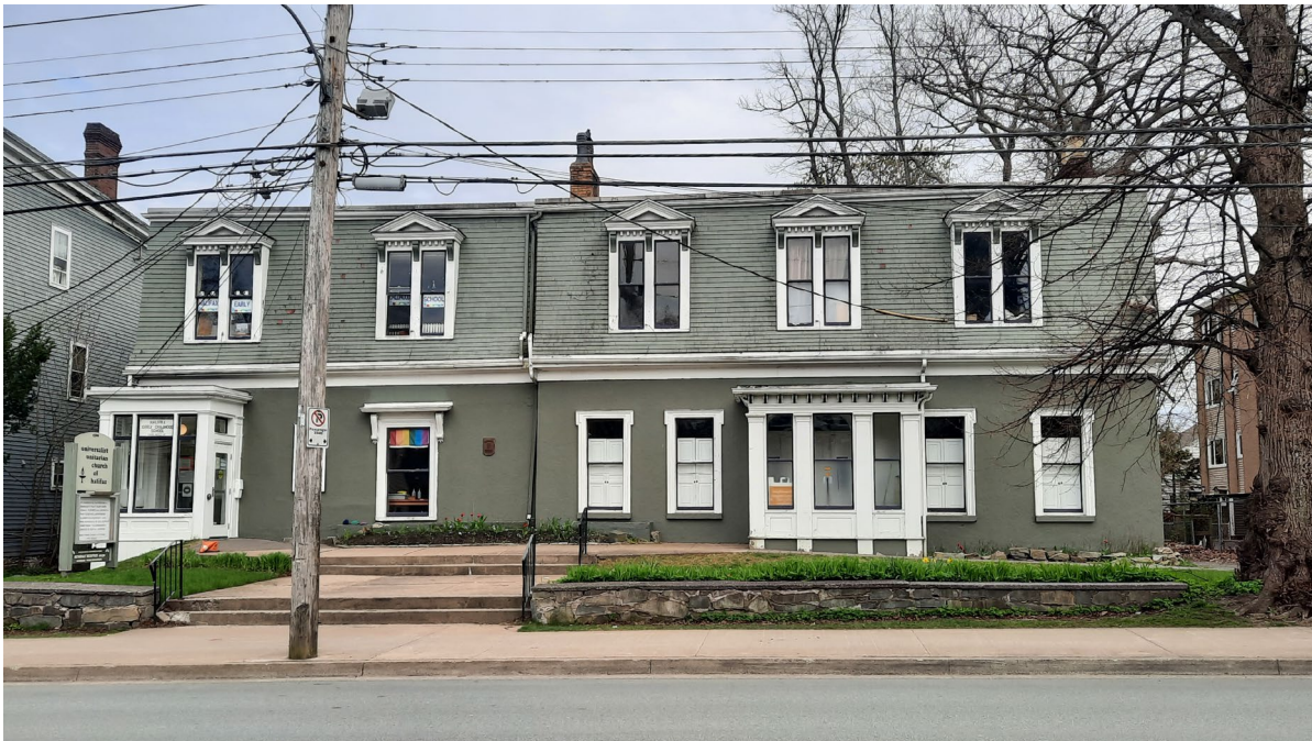
Figure 5: North façade of 5500 Inglis Street (May 4, 2021)
