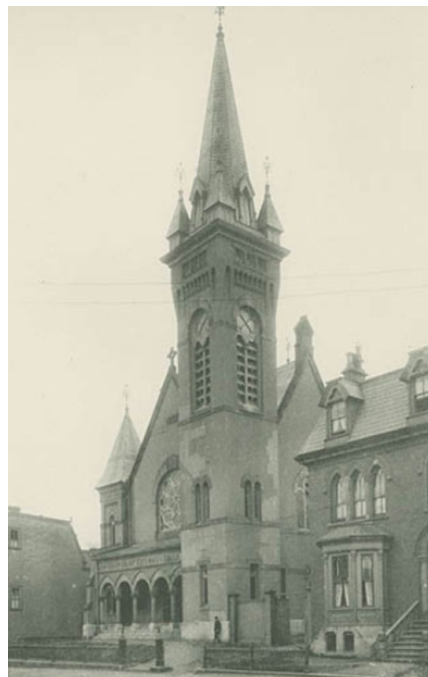
Figure 3: Former Brunswick Street Location of the Church of the Redeemer, 1899 (Source: Nova Scotia Archives O/S F107 H13 C23)
