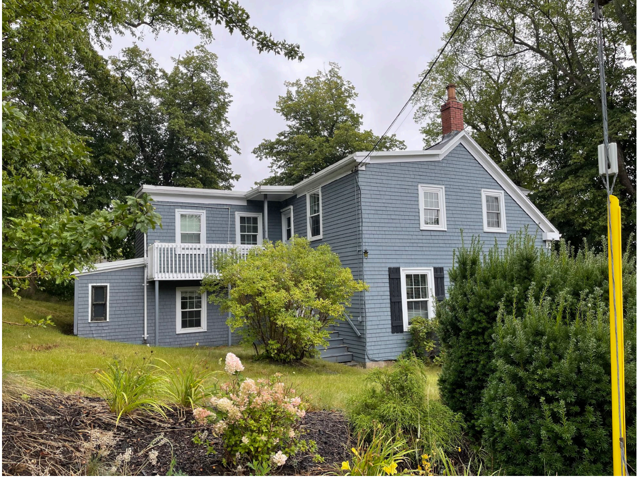
Figure 19: Western elevation of 1262 Bedford Highway (August 30, 2021)
