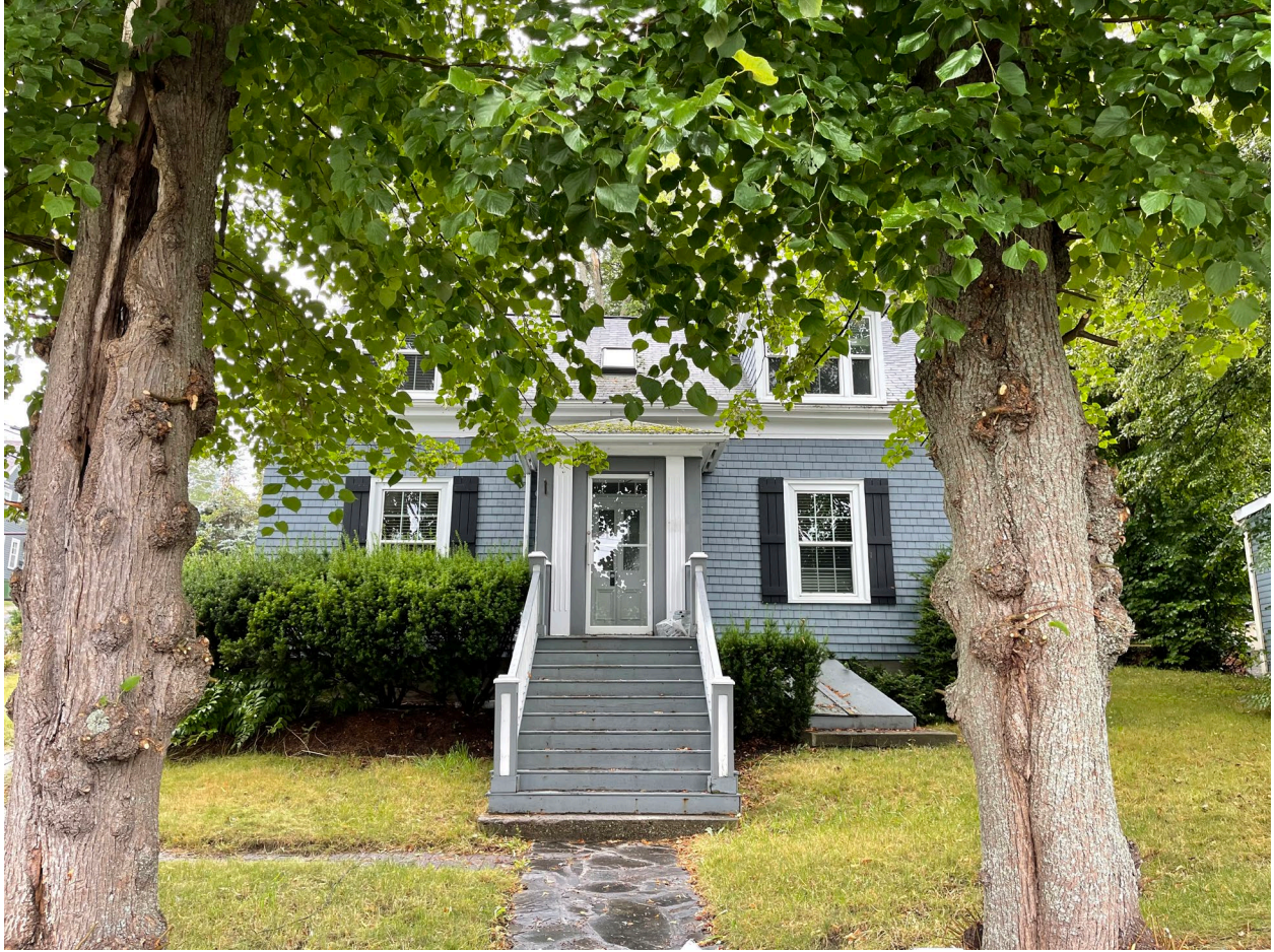
Figure 15: Southeast [front] elevation of 1262 Bedford Highway (August 30, 2021)
