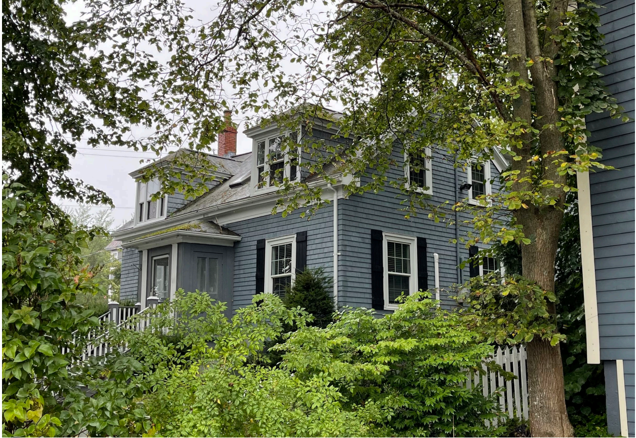
Figure 16: Eastern elevation of 1262 Bedford Highway (August 30, 2021)
