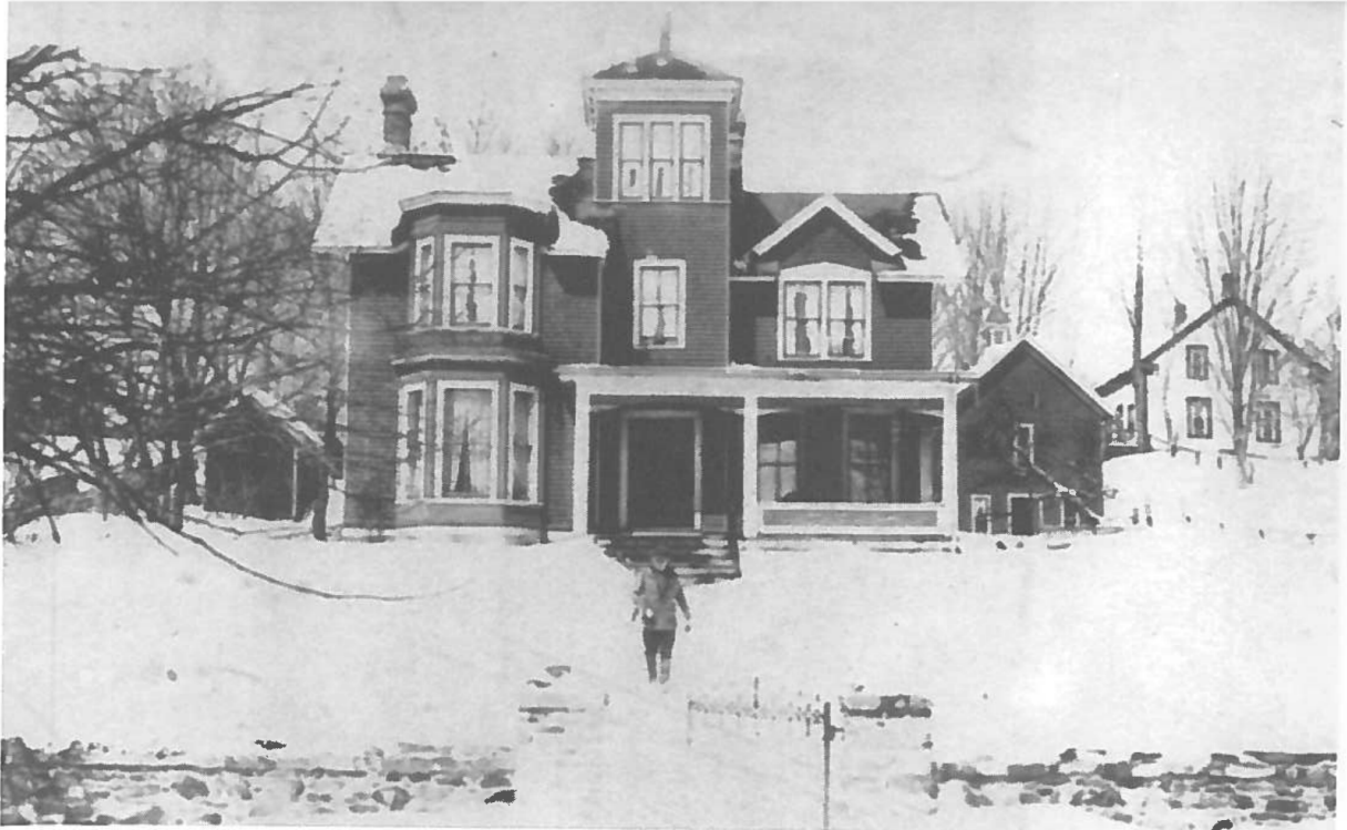
Figure 31: Gypsy Hill [Demolished], former home of J.E. DeWolf, located across Meadowbrook Drive from Honeycote (Tony Edwards, 2007)
