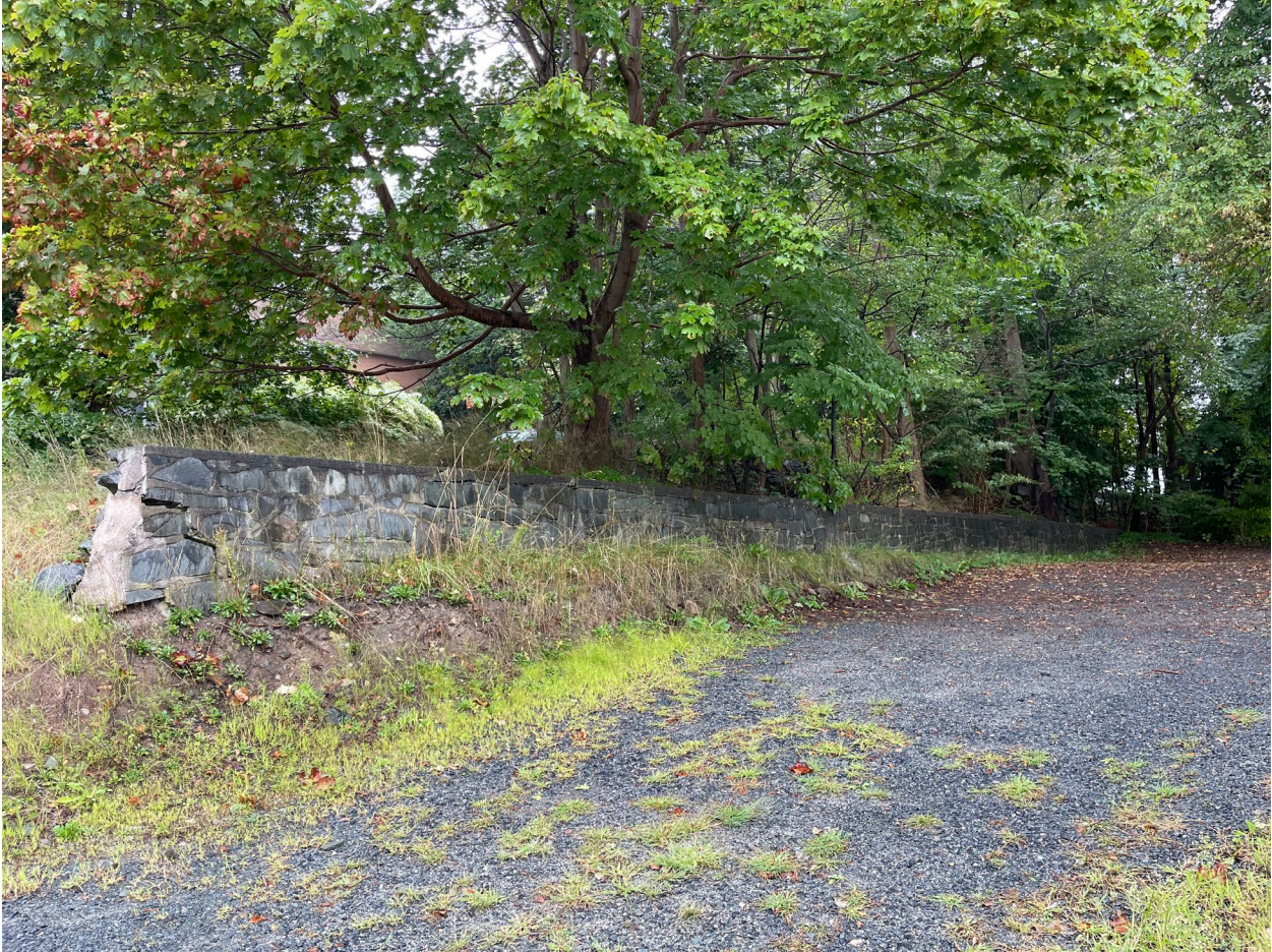
Figure 27: Retaining wall in the rear of 1262 Bedford Highway approximately showing the rear boundary line shared with “Lot A” which was sold off separately in 1960 (August 30, 2021)
