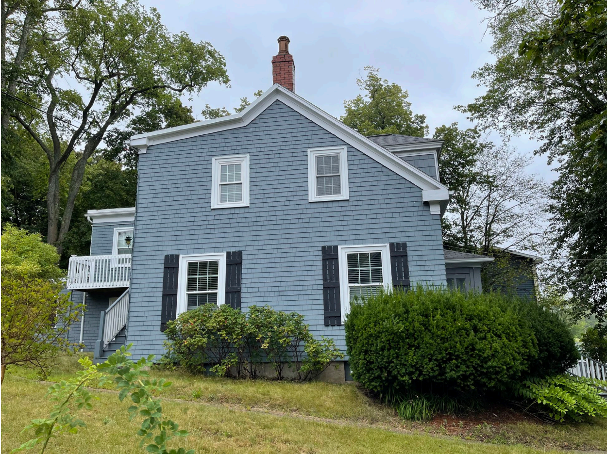
Figure 18: Southwest elevation [Meadowbrook Drive] of 1262 Bedford Highway (August 30, 2021)
