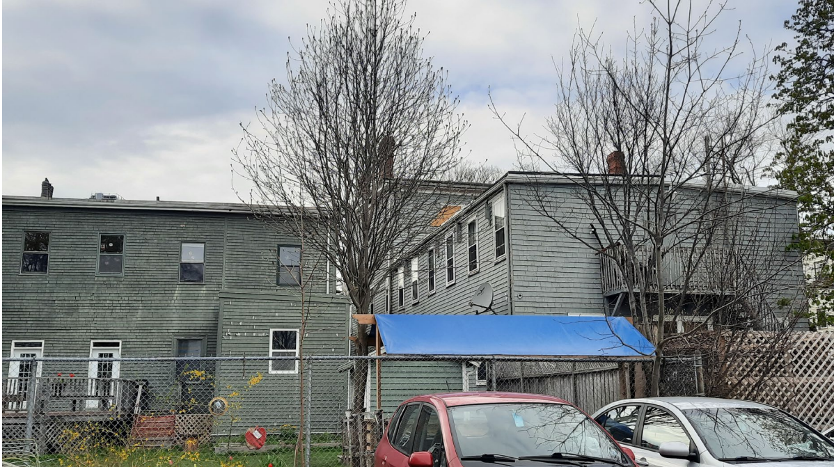
Figure 19: West exterior wall of 5492 Inglis Street (right; May 4, 2021)
