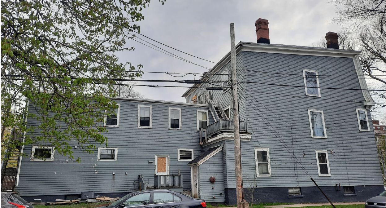
Figure 17: East and south exterior walls of 5492 Inglis Street (May 4, 2021)
