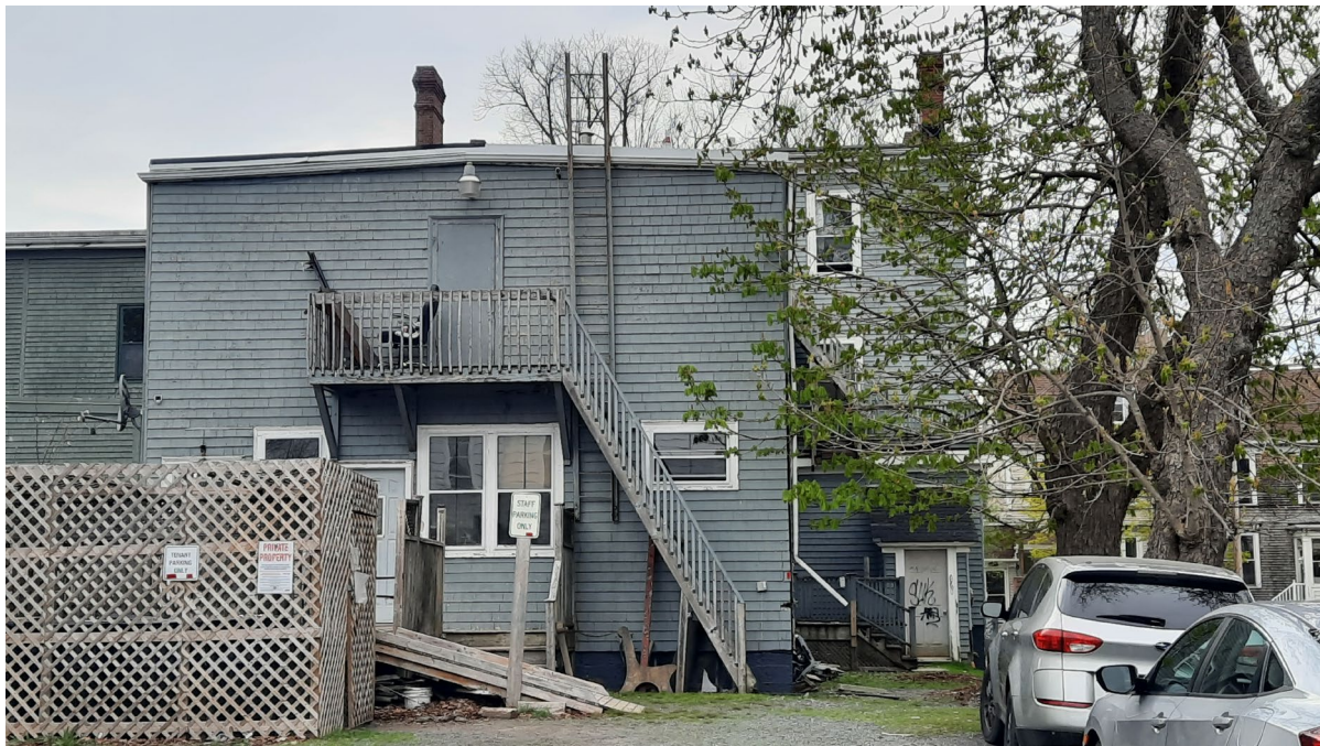
Figure 18: South (rear) exterior wall of 5492 Inglis Street (May 4, 2021)
