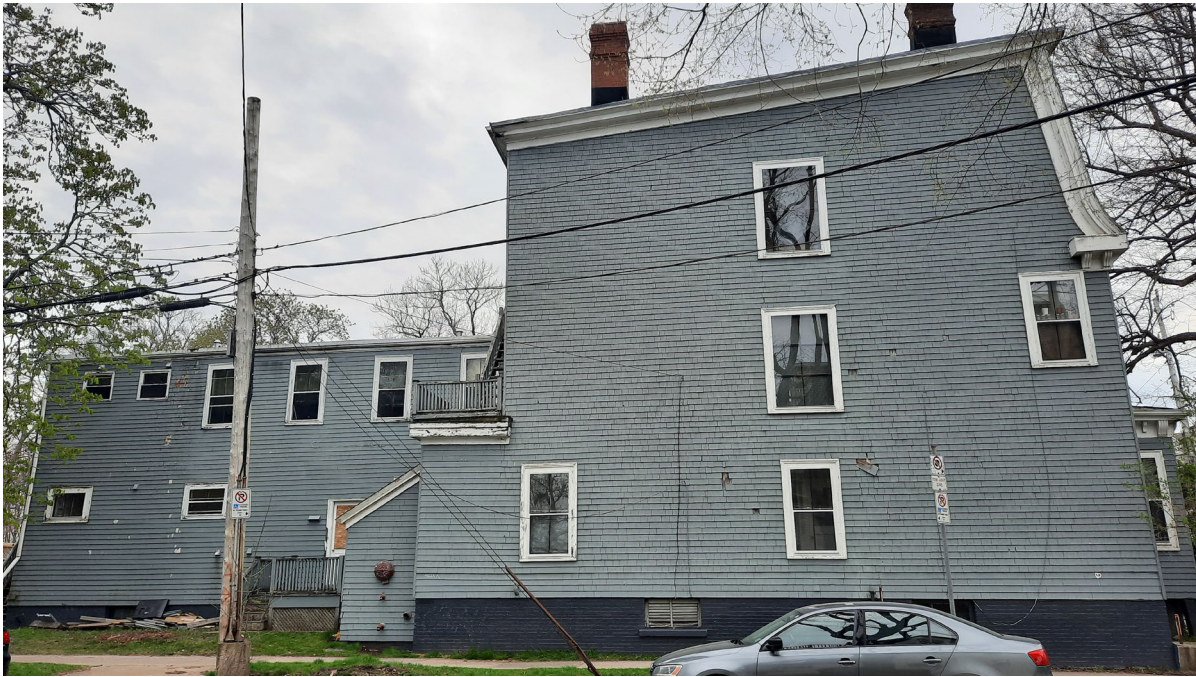
Figure 16: East (South Bland) façade of 5492 Inglis Street (May 4, 2021)
