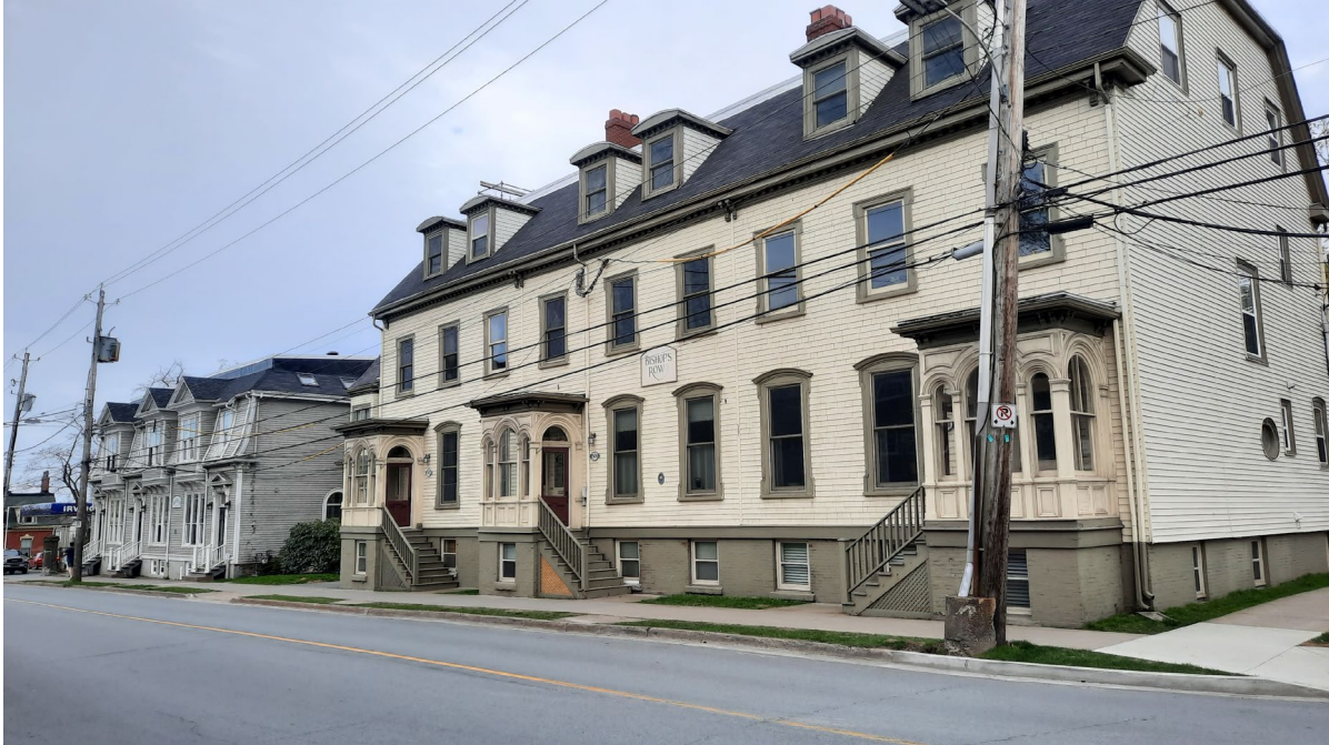
Figure 22: Neighbouring properties to the east of 5492 Inglis Street (May 4, 2021)
