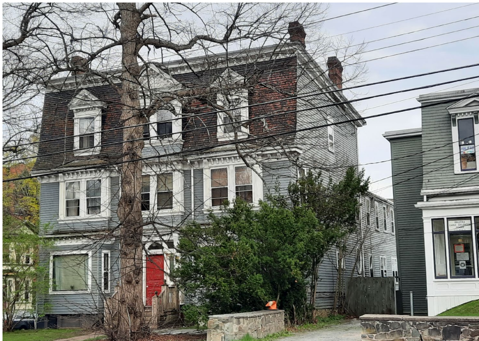
Figure 20: North (Inglis) façade of 5492 Inglis Street (May 4, 2021)
