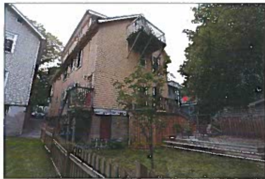
③ VIEW OF EAST & SOUTH SIDE
