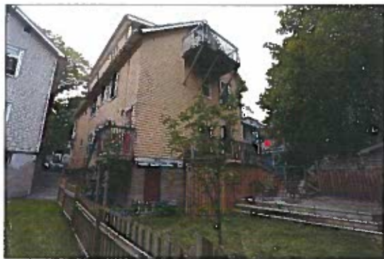
③ VIEW OF EAST & SOUTH SIDE
