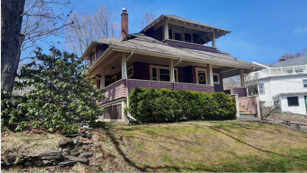
Figure 6: Front and west wall of 173 Crichton Avenue (April 9, 2021)
