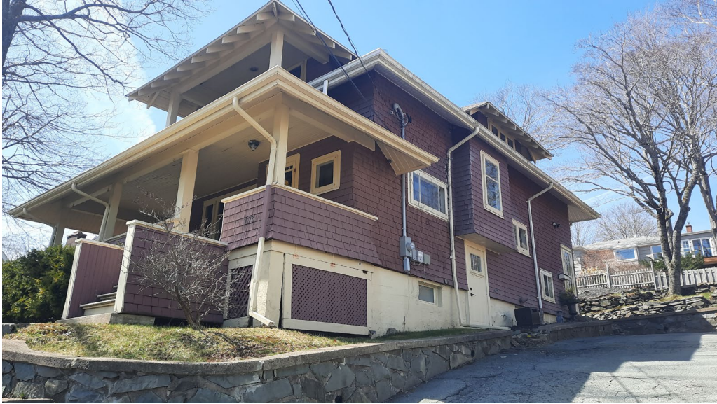
Figure 10: Front and west wall of 173 Crichton Avenue (April 9, 2021)
