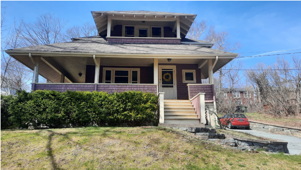
Figure 5: Façade of 173 Crichton Avenue (April 9, 2021)
