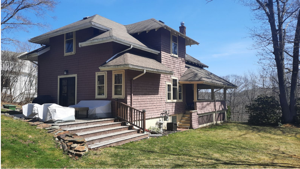
Figure 8: West and north (rear) walls of 173 Crichton Avenue (April 9, 2021)
