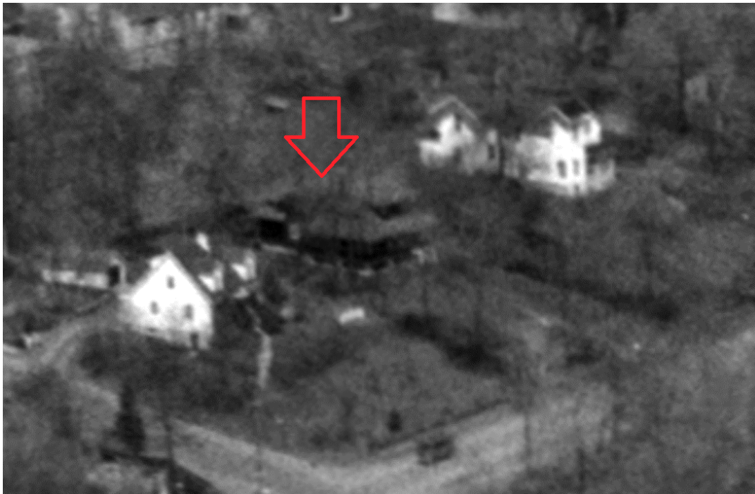
Figure 11: Aerial imagery of Crichton Avenue circa 1969, with the subject property identified in red (Source: Halifax Municipal Archives 101-80C-1-6.23)
