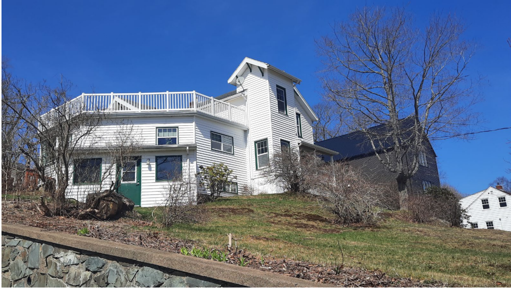
Figure 13: 175 Crichton Avenue (formerly 177 Crichton Avenue; Charles J. Keeler's house) as visible from the driveway of the subject property (April 9, 2021)
