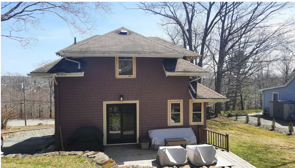
Figure 9: North (rear) wall of 173 Crichton Avenue (April 9, 2021)
