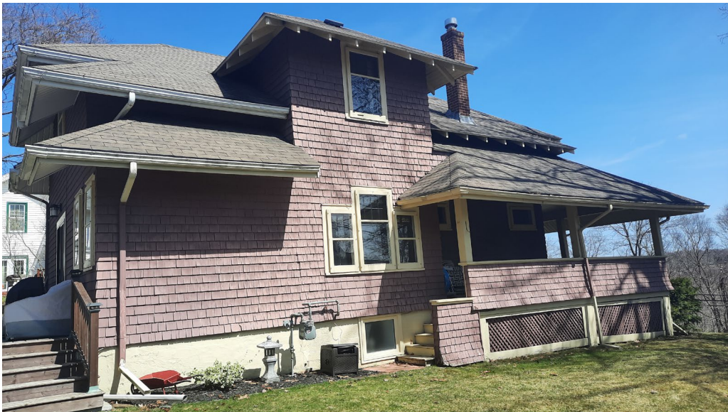
Figure 7: West wall of 173 Crichton Avenue (April 9, 2021)
