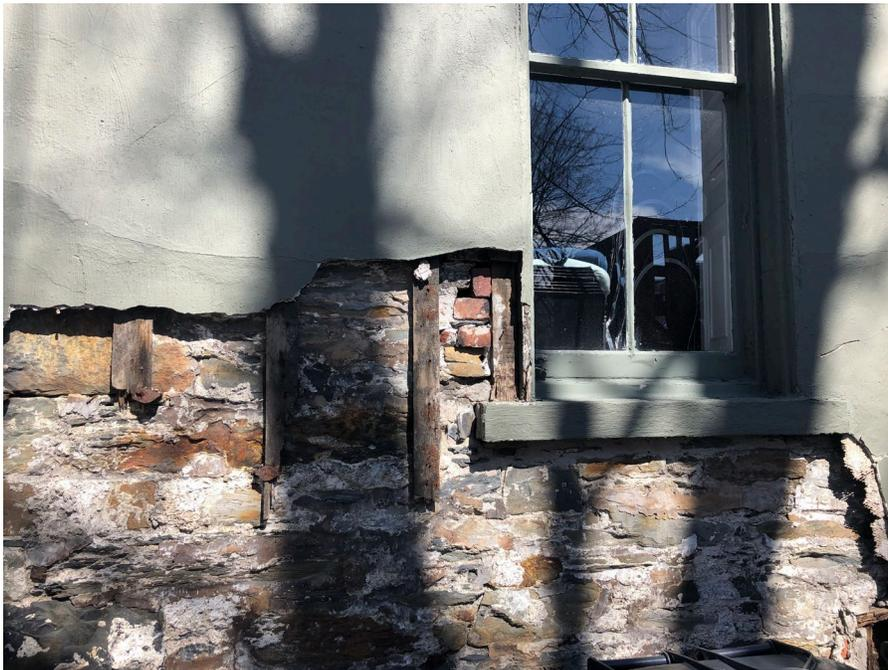
Figure 10: Evidence of original rubble stone walls underneath stucco cladding on south façade (April 9, 2021)
