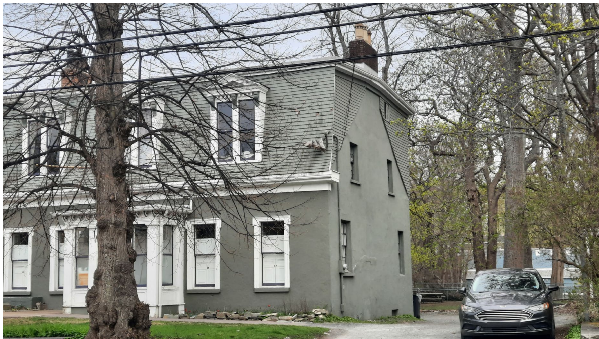
Figure 12: Evidence of original gable roofline on the west facade (May 4, 2021)
