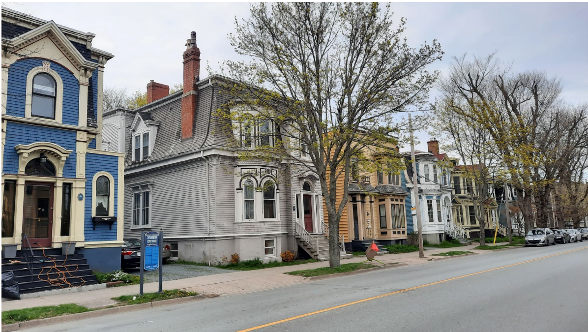
Figure 13: Inglis Street Heritage Streetscape at 5651-5691 Inglis Street (May 4, 2021)
