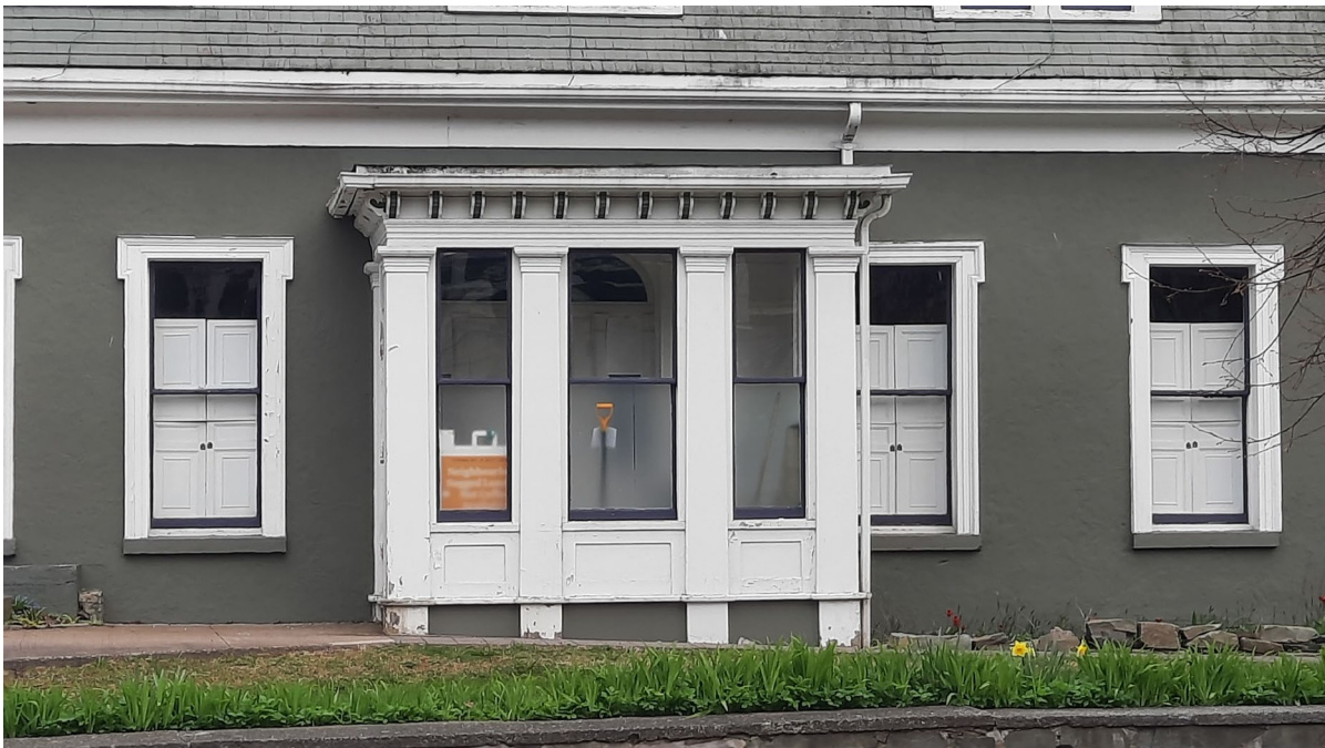
Figure 9: Storm porch entrance with piers, wood panelling and bracket detailing (May 4, 2021)
