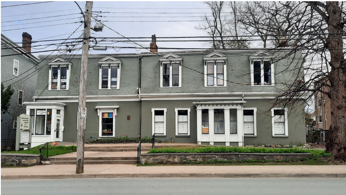
Figure 5: North façade of 5500 Inglis Street (May 4, 2021)
