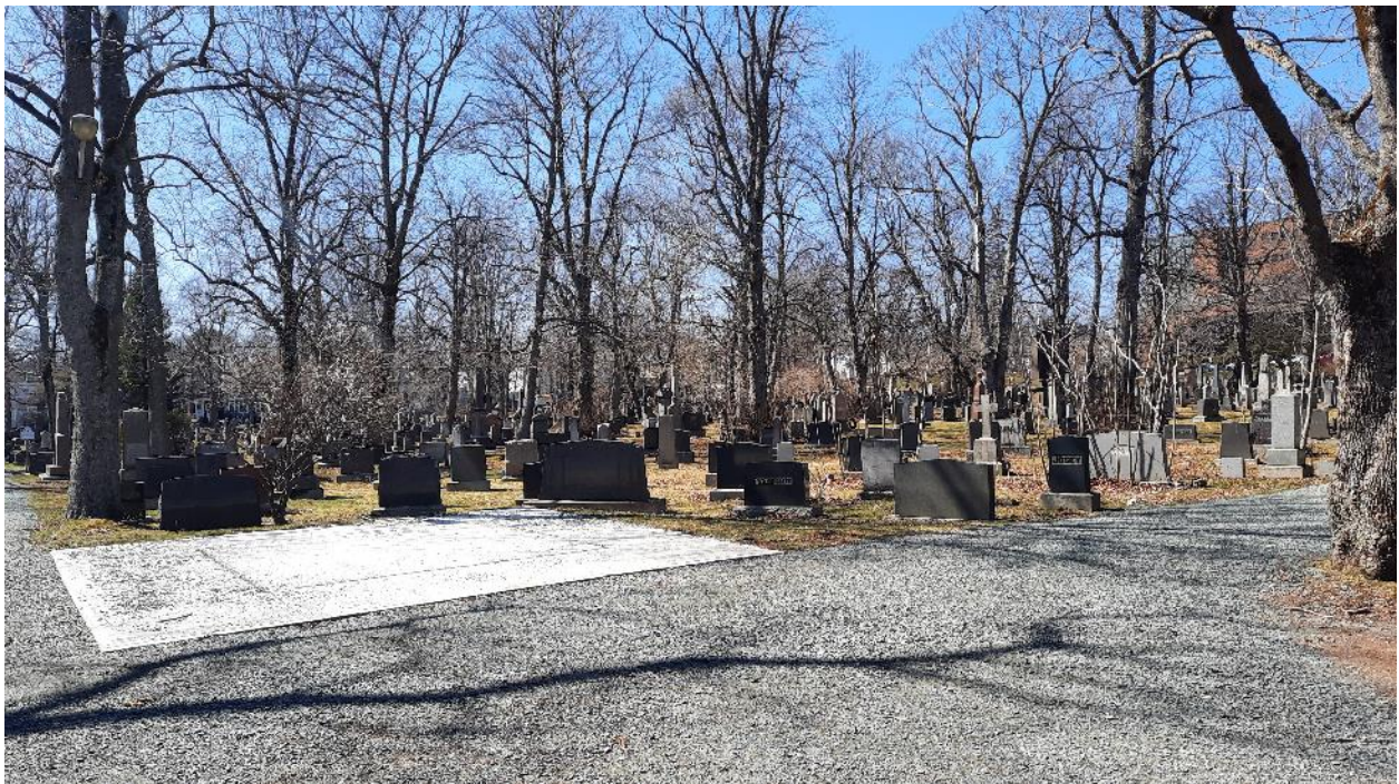
Figure 14: Concrete pad for future columbarium site
