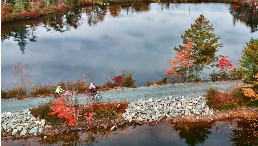
Gaetz Brook Greenway - Construction finished in 2020 by SATA Trails Society
