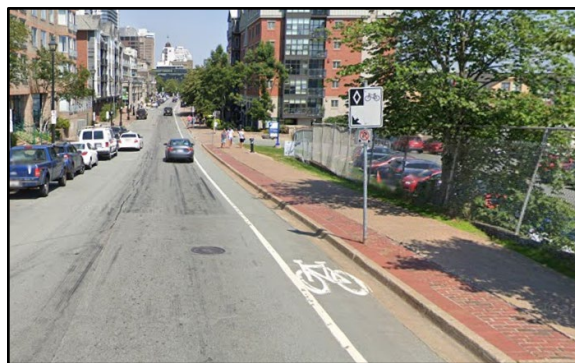
Figure 2.2.2: Painted bike lane on Lower Water Street
