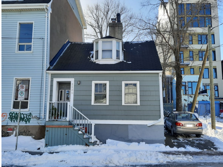
Figure 7: North façade of 2224 Maitland Street (09 February 2021)
