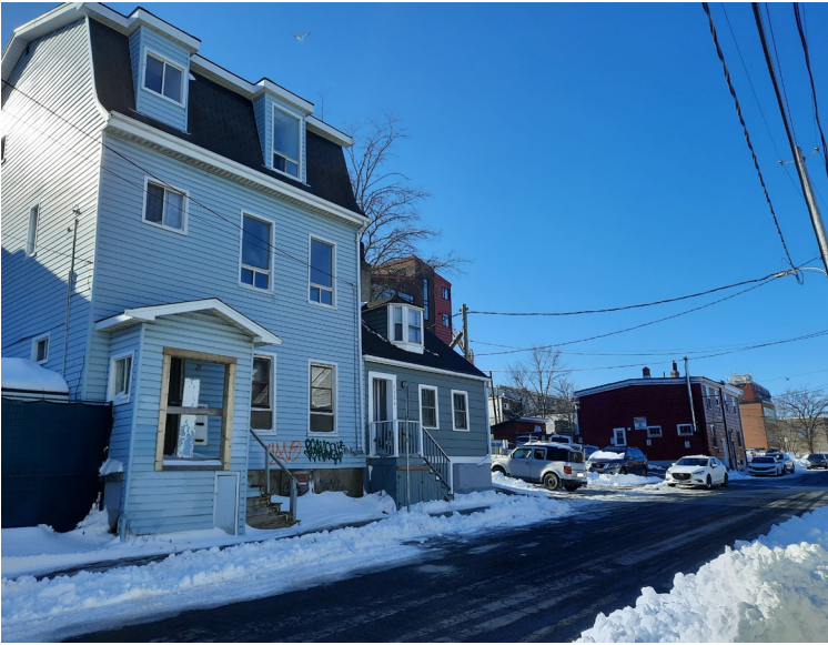
Figure 9: Maitland Street facing north from the intersection with Cornwallis Street (09 February 2021)
