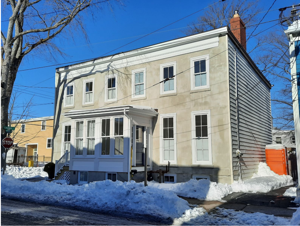
Figure 9: West and south façades of 2379-2381 Moran Street (09 February 2021)
