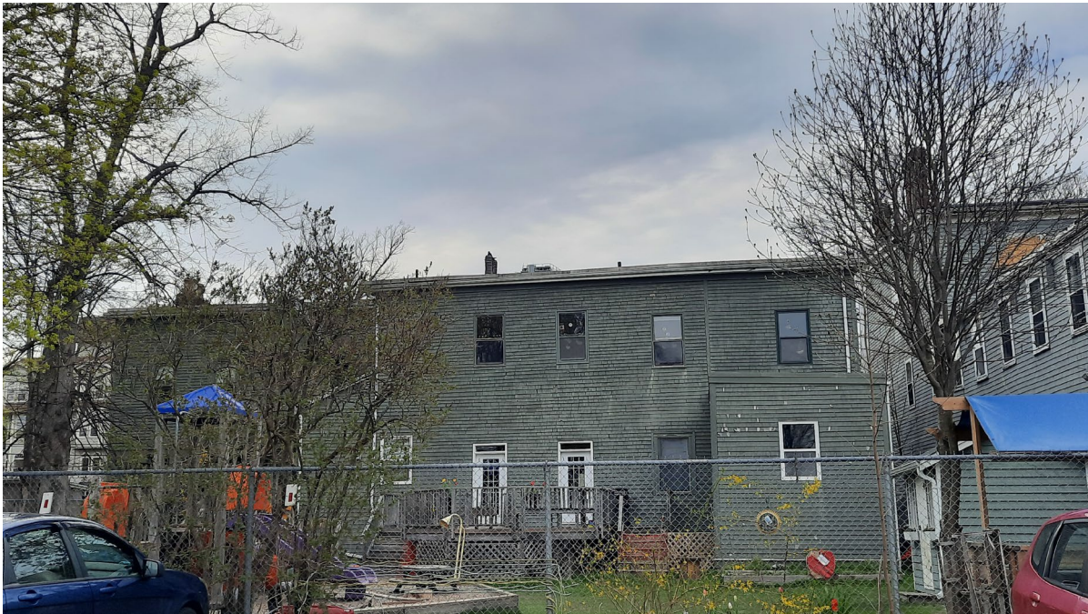
Figure 7: South façade of 5500 Inglis Street (May 4, 2021)
