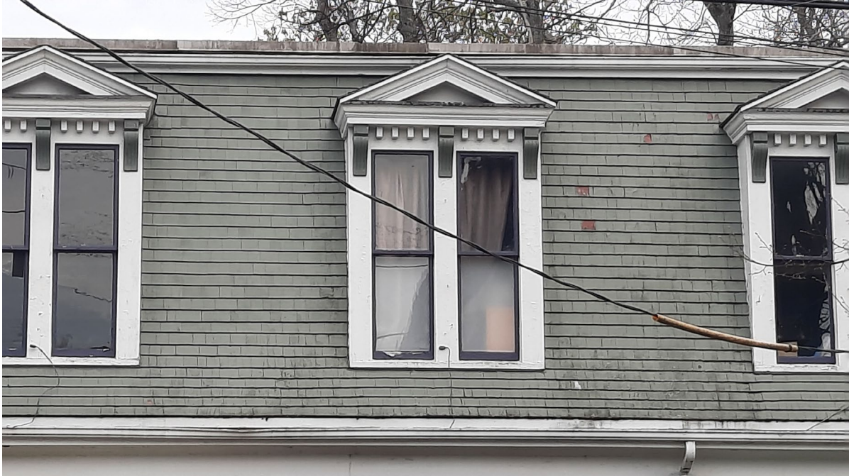
Figure 8: Dormers with pediment style roof, dentils and corbels (May 4, 2021)
