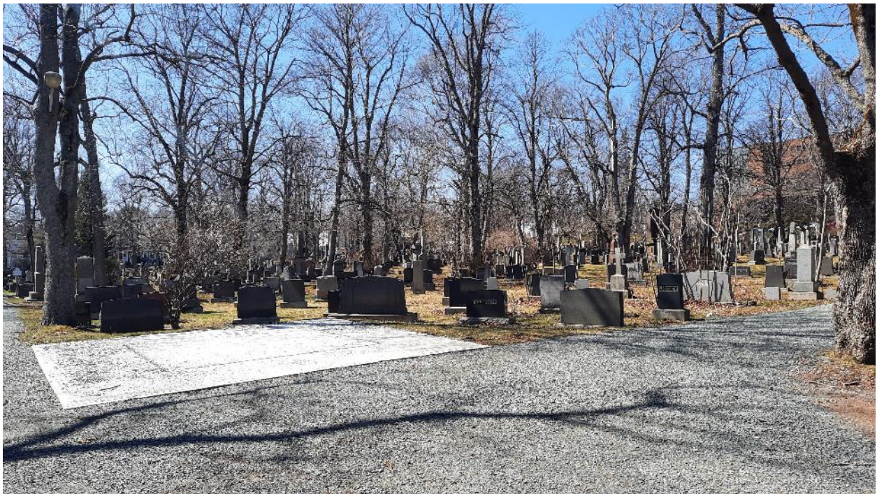
Figure 14: Concrete pad for future columbarium site
