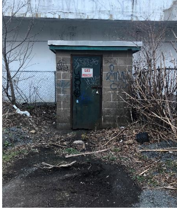
Figure 19: Gas House to the west of the tool shed (23 April 2021)
