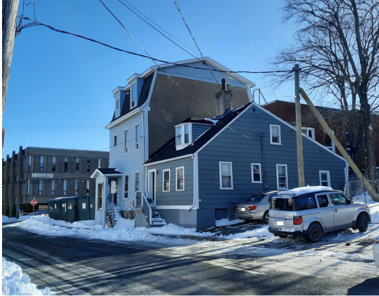
Figure 10: Maitland Street facing south from 2221 Maitland Street (09 February 2021)
