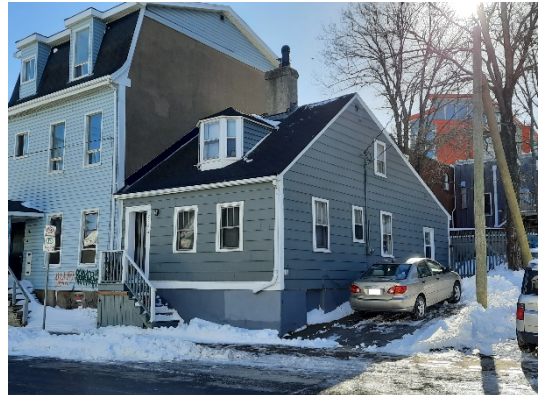
Figure 1: 2224 Maitland Street Staff Site Visit (09 February 2021)
