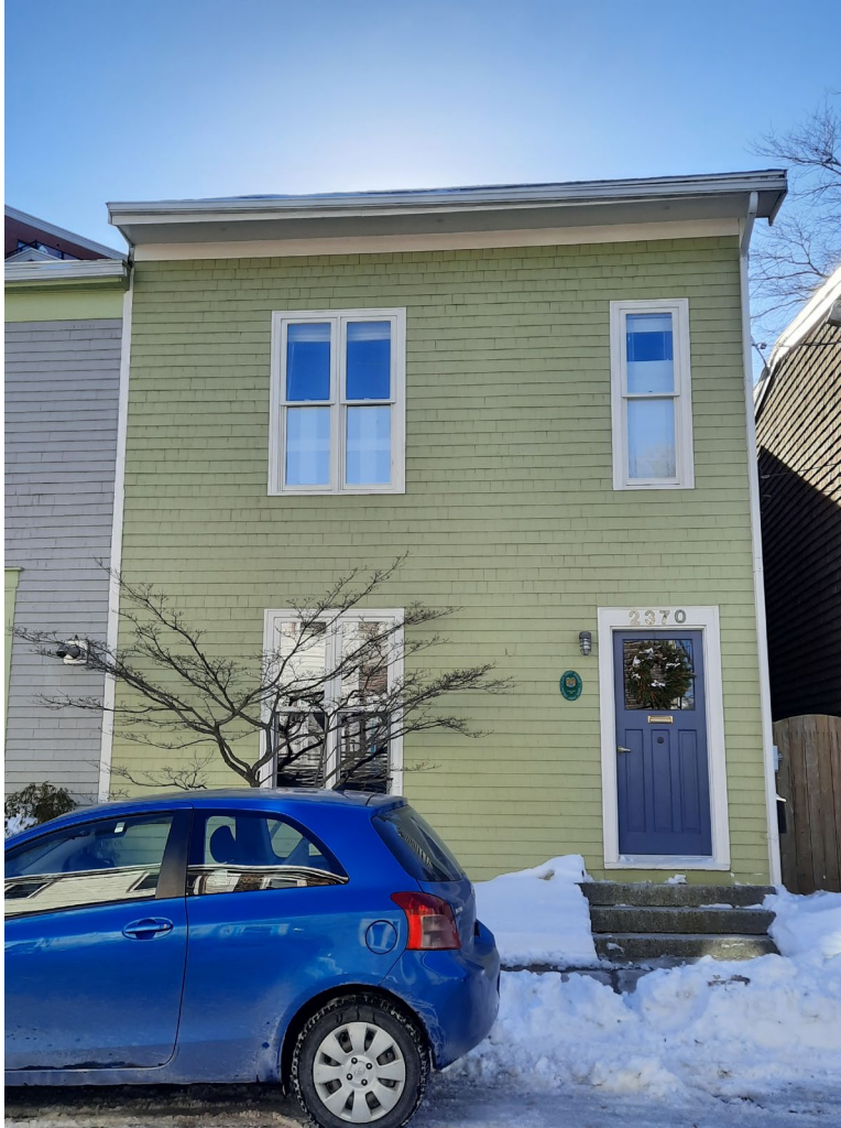
Figure 16: Registered Heritage Property at 2370 Moran Street (09 February 2021)
