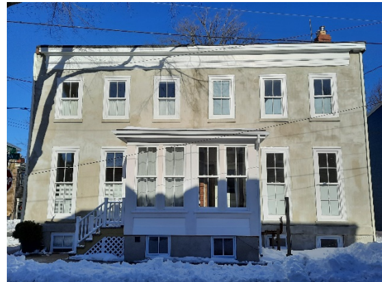
Figure 1: 2381 Moran Street (left) Staff Site Visit (09 February 2021)
