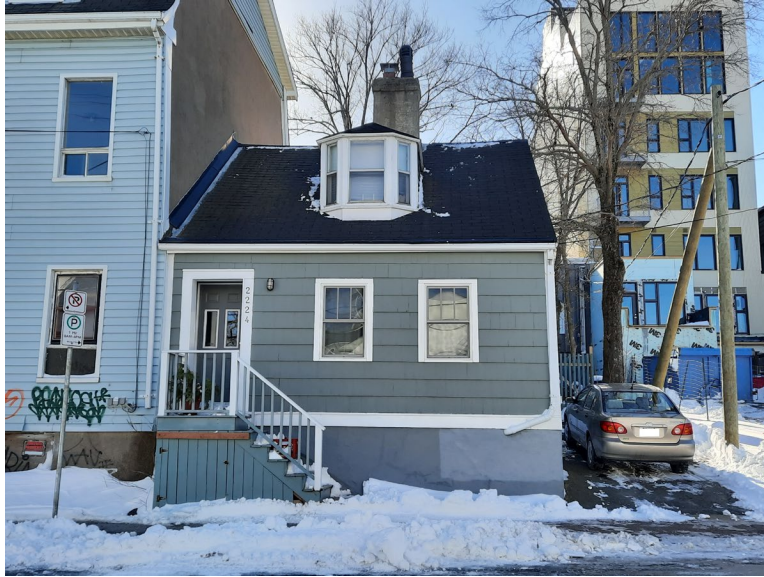
Figure 7: North façade of 2224 Maitland Street (09 February 2021)
