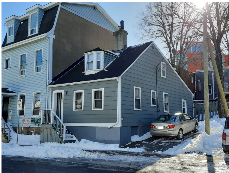
Figure 8: North and west façades of 2224 Maitland Street (09 February 2021)
