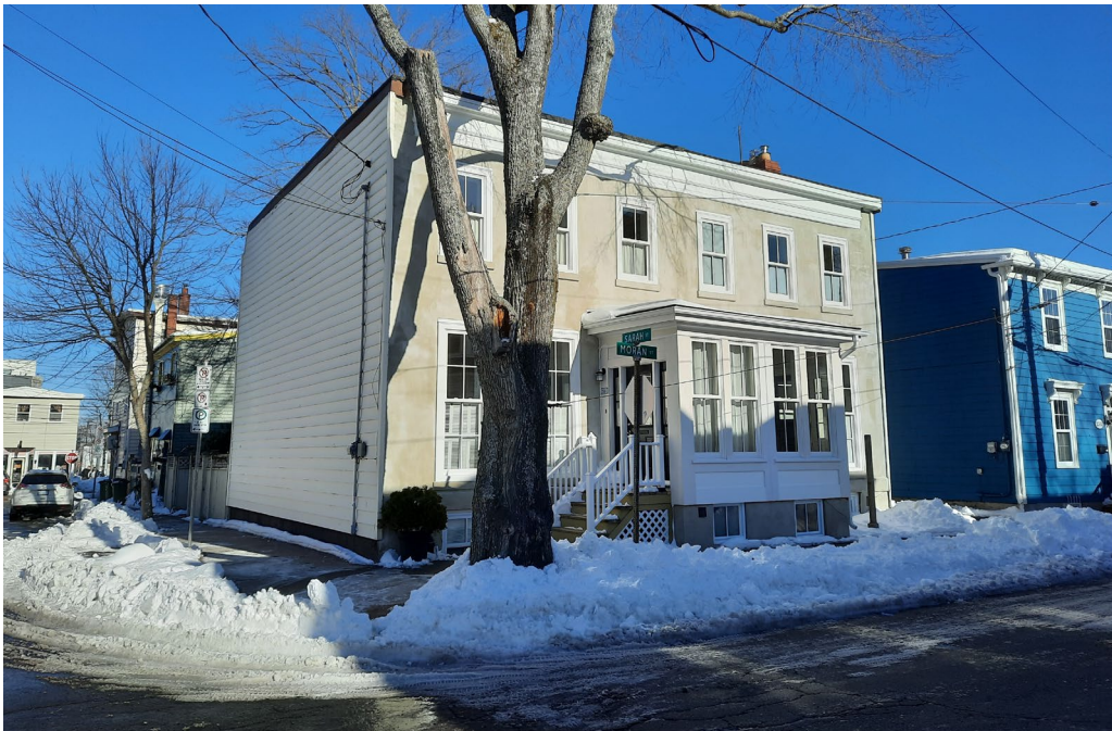
Figure 10: West and north façades of 2379-2381 Moran Street (09 February 2021)
