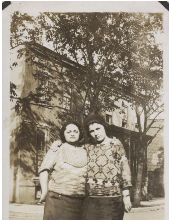
Figure 12: 2381 Moran Street circa 1923 (Source: 2381 Moran Street Property Owners)
