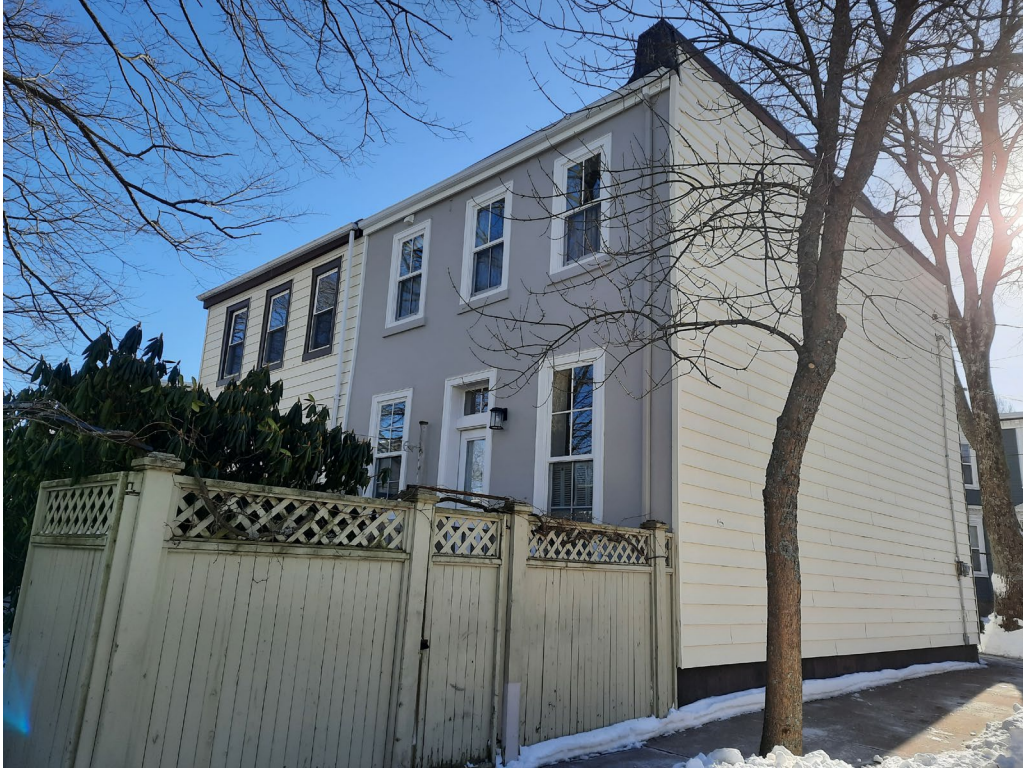
Figure 11: East and north facades of 2381 Moran Street (09 February 2021)
