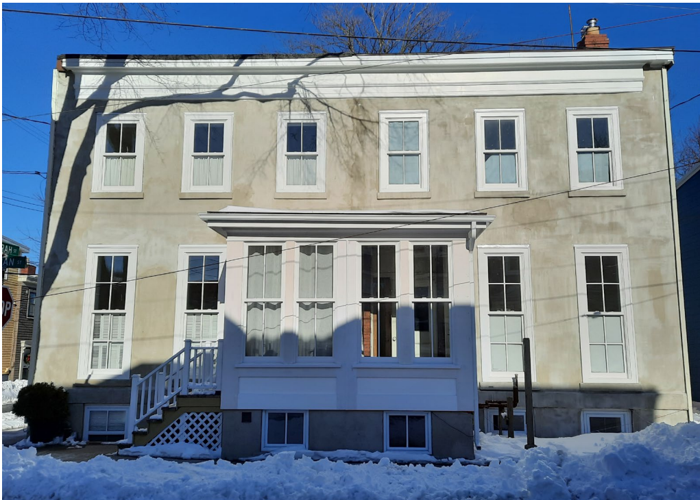
Figure 8: West facade of 2379-2381 Moran Street (09 February 2021)
