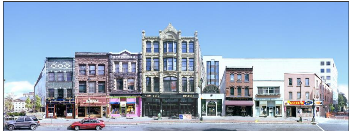
Commercial Block in the Barrington Street Area
