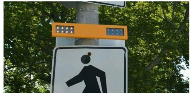
RRFBs are pedestrian activated crosswalk systems which consist of two rapidly and alternately flashing rectangular amber beacons mounted above the side mounted pedestrian crossing signs. RRFBs can enhance safety at unsignalized intersections and mid-block pedestrian crossings by increasing driver awareness of potential pedestrian conflicts and by improving driver yielding behavior.
