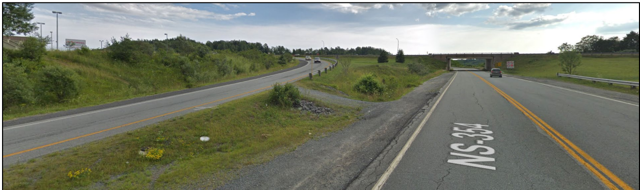
Figure 1: Crossing Location of Beaver Bank Connector and Highway 101 Off-ramp (Exit 2)
