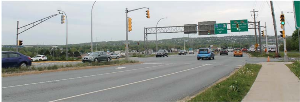
Photo 2 – Portland Street and Site Access #2/NS Highway 111 Southbound Onramp
