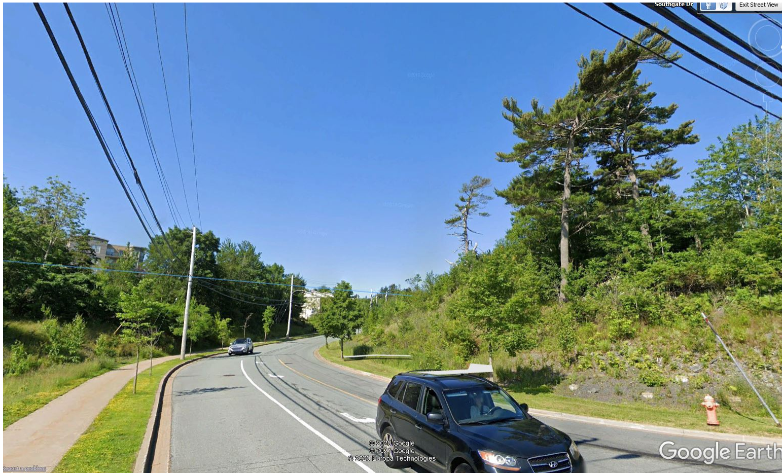
Subject site BH-1 seen from the intersection of Southgate Drive and Bedford Highway
