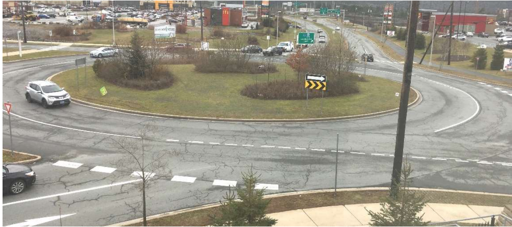
Photo 3: Looking west on Larry Uteck Blvd at Nine Mile Drive
