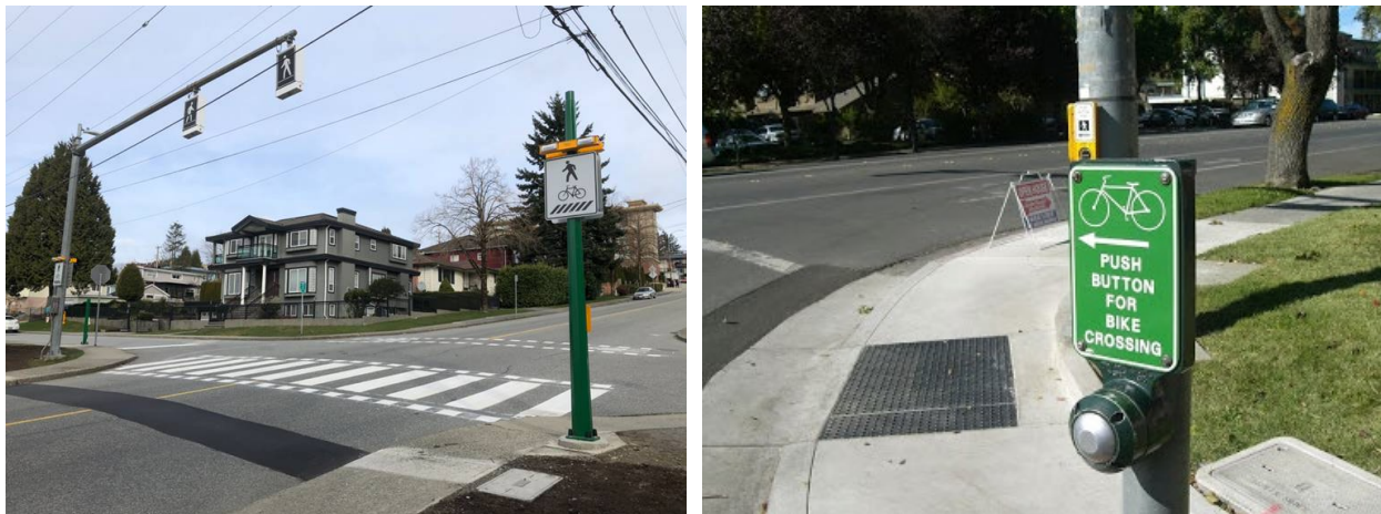
From left to right: Figure 6: Sample Image of Pedestrian and Cyclist Activated RRFB from Burnaby BC (future desired treatment); Figure 7: Close-Up of Cyclist Push Button (upgrade required in future pending legislation changes)
