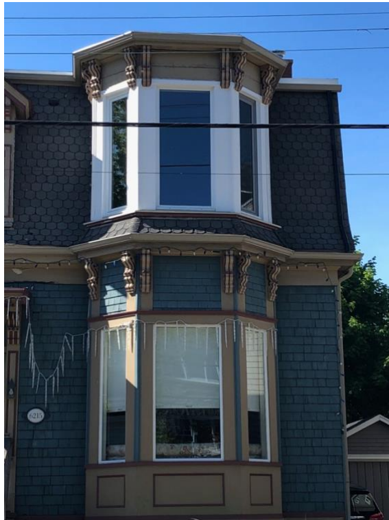
Figure 19: Two-storey bay window on the south façade
