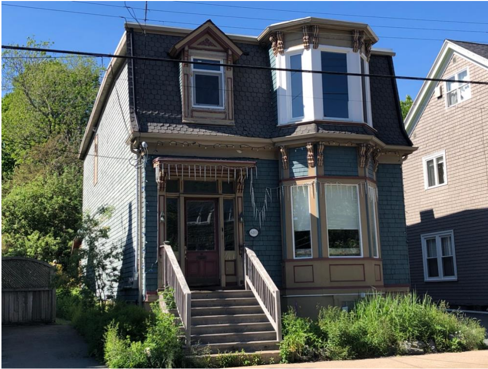
Figure 12: South and west façades
