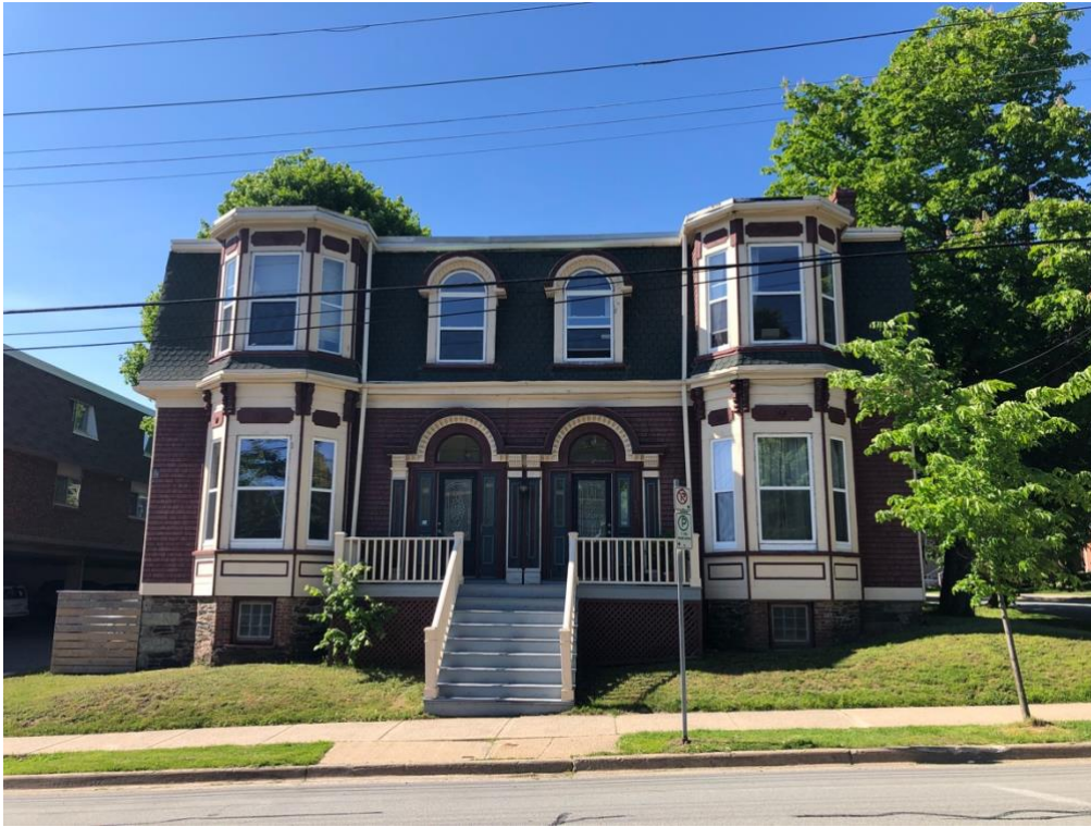
Figure 16: Second Empire style house at 6247-49 Coburg Road
