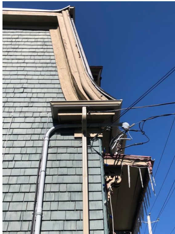
Figure 17: Mansard roof with returned eaves
