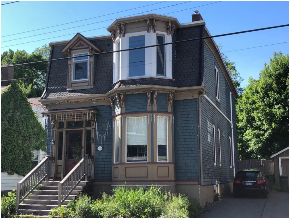
Figure 13: South and east façades
