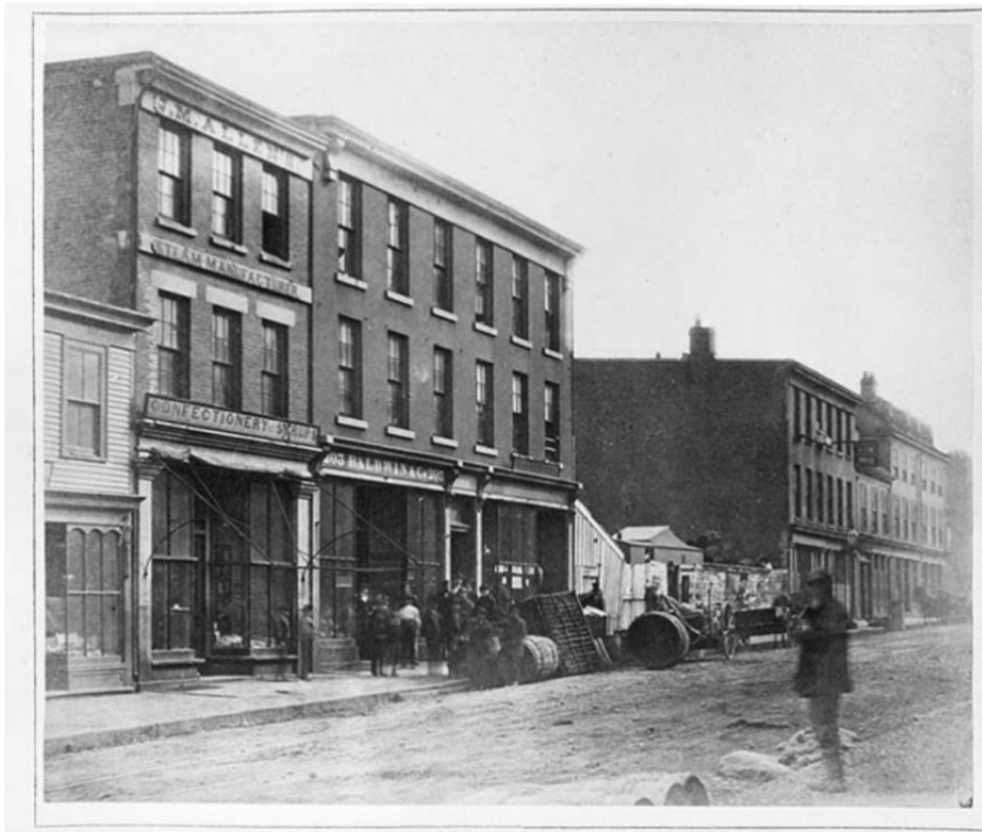
Figure 9: Baldwin & Co. on Barrington Street, undated (Source: Nova Scotia Archives)
