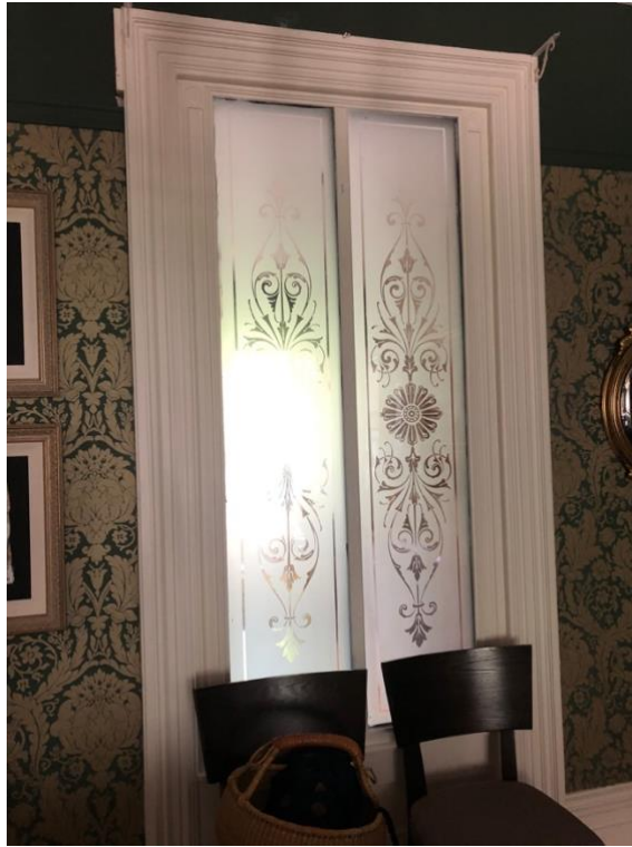
Figure 28: Acid etched window between the dining room and northeast addition
