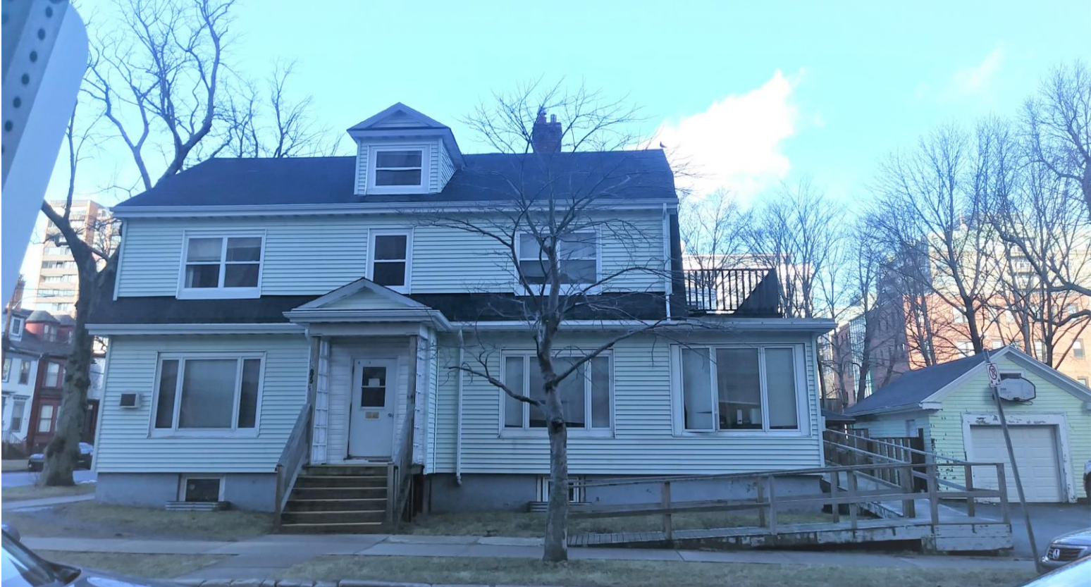
Subject site seen from College Street
