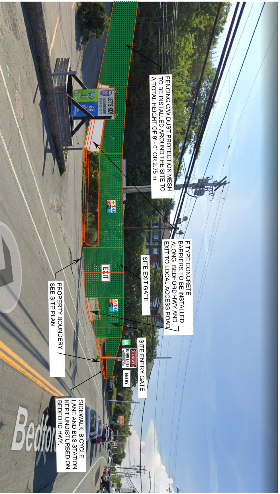
FENCING CW DUST PROTECTION MESH TO BE INSTALLED AROUND THE SITE TO A TOTAL HEIGHT OF 9' - 0" OR 2.75 m
